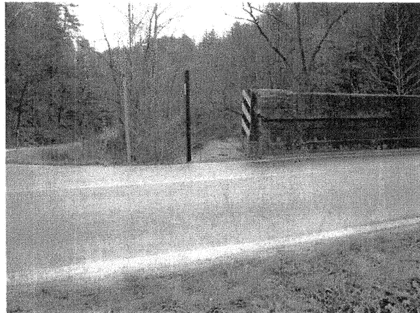
Photograph No. 12: This photograph was taken from 6' left of the -L- alignment, looking east, across proposed End Bent No. 2.
