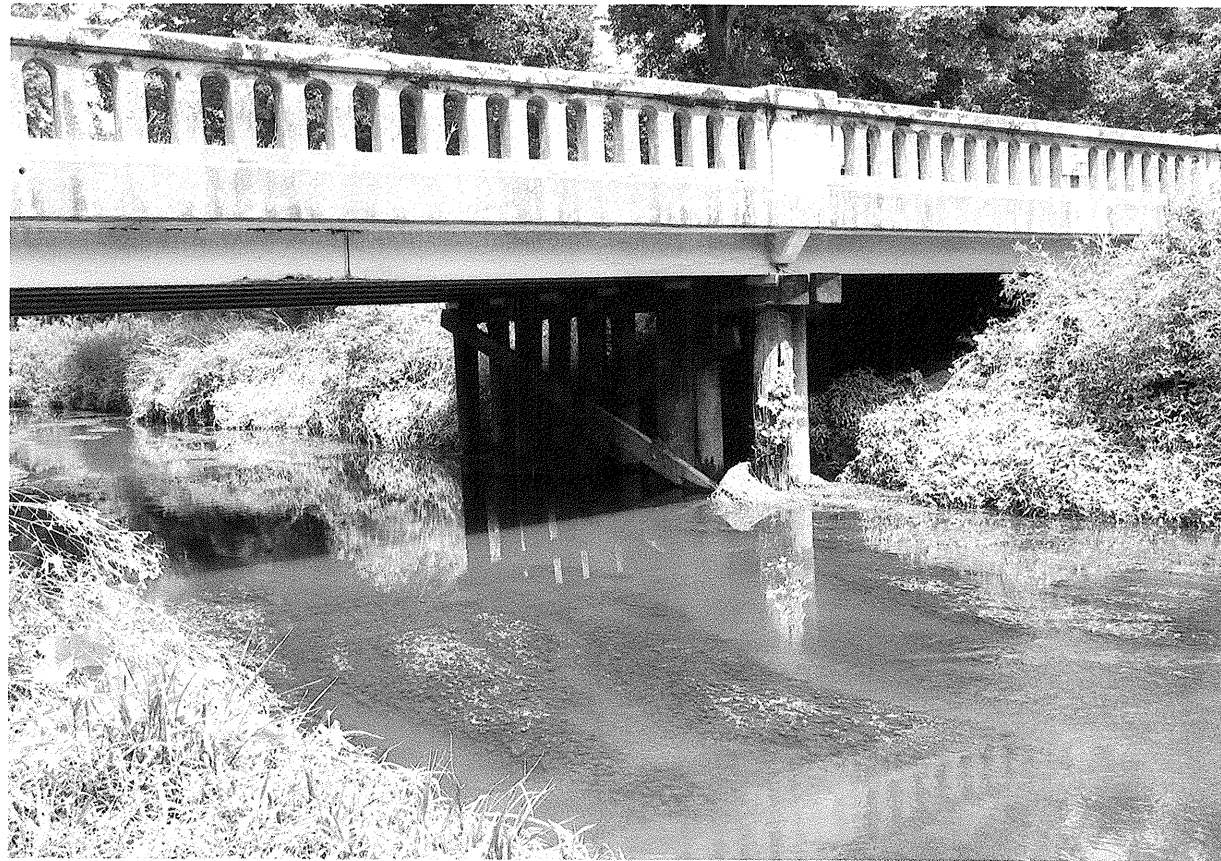
Bridge No.53 from EB1 looking Northeast
