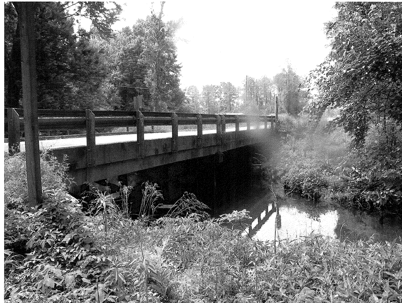
Looking South Toward End Bent 1
