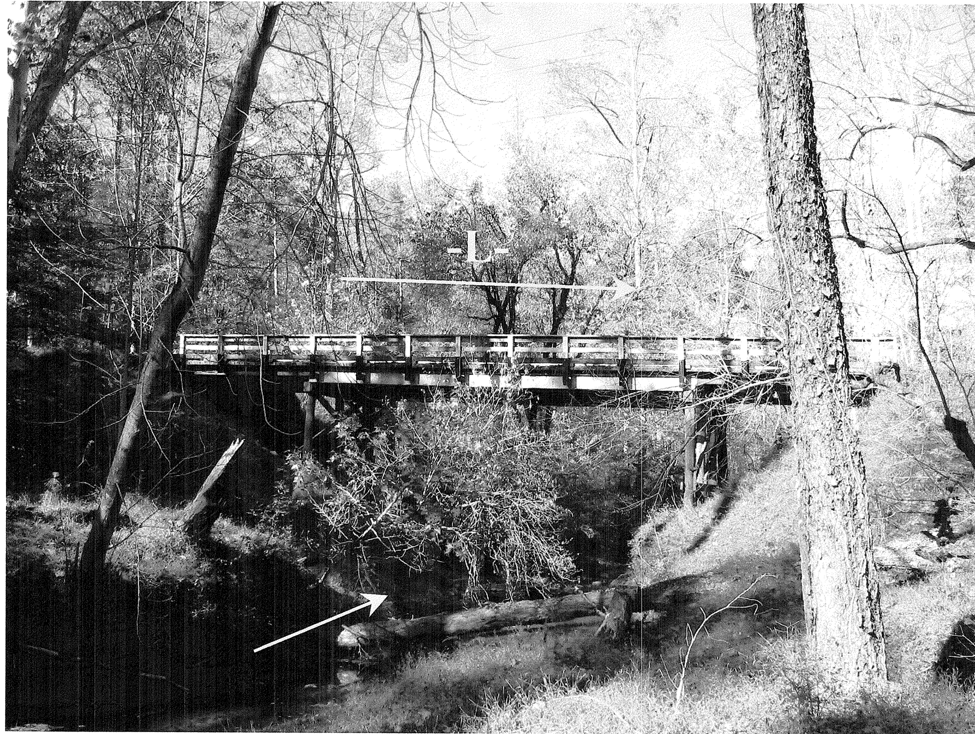
Bridge No. 158 on -L- (SR 1402) over a Creek
