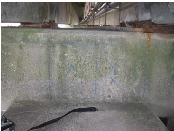
Bent 187: bent cap, north face
