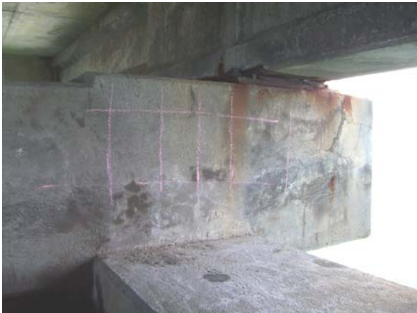
Bent 177: north elevation, west end
