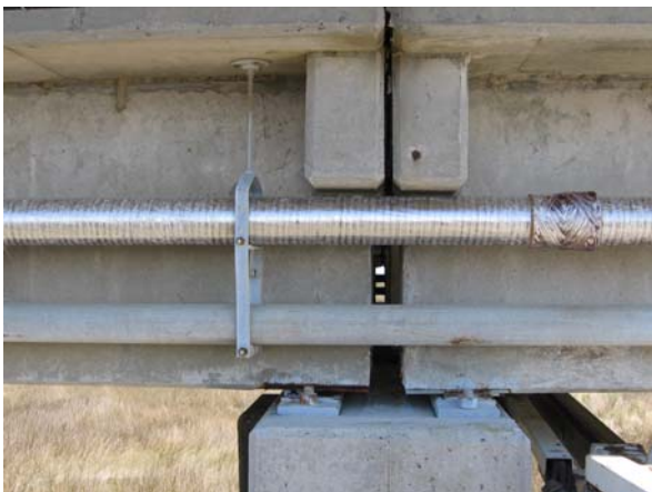
Bent 88: Girder ends and bearing, west side
