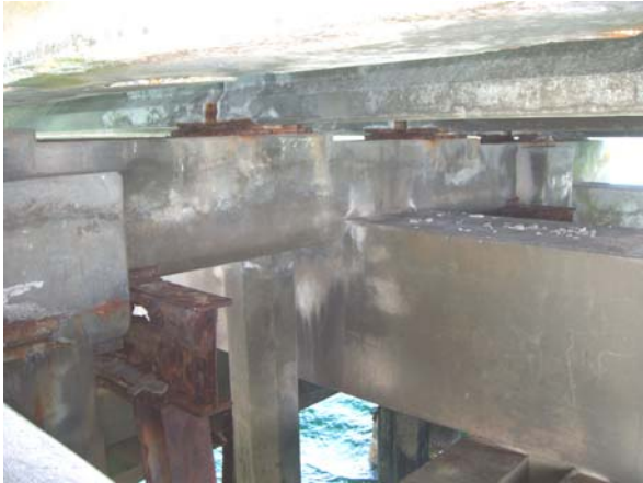
Bent 187: south elevation
