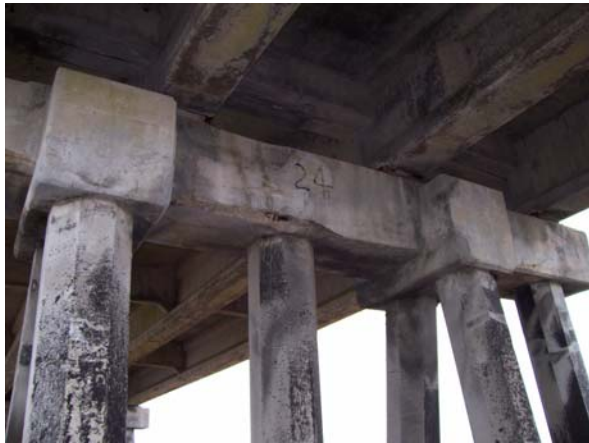
Bent 24: large SP
