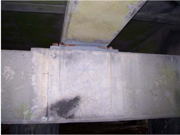
Bent 3, bent cap: SP south elev
