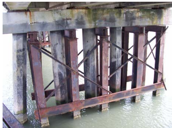
Bent 117: north elevation
