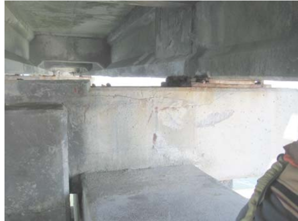
Bent 164, Bent cap: south face
