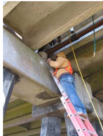
Bent 12: Bent cap, south face
