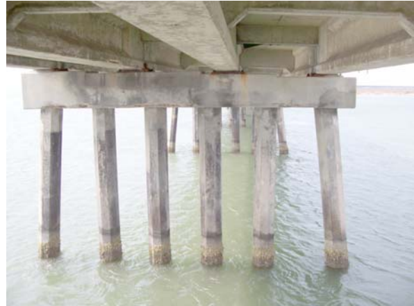
Bent 103: south elevation
