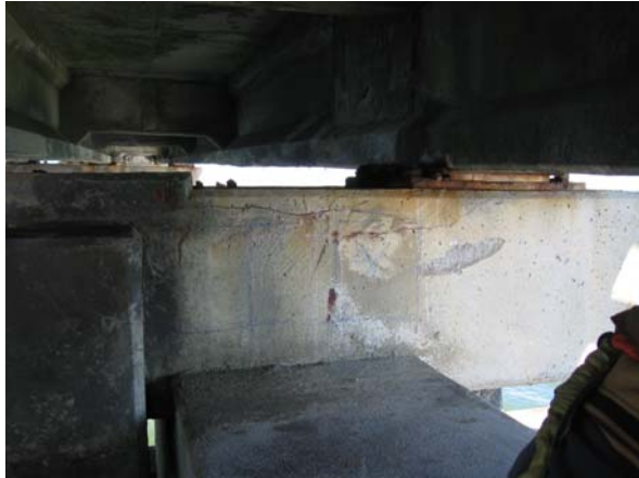
Bent 164, Bent cap: south face
