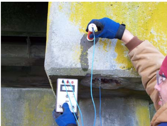
Bent 193: east end
