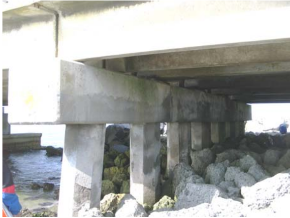
Bent 201: south elevation
