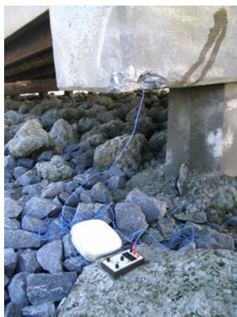
Bent 201: north elevation
