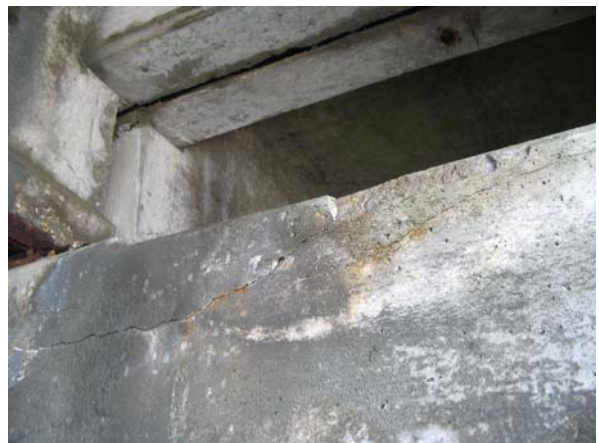
Bent 201: north elevation
