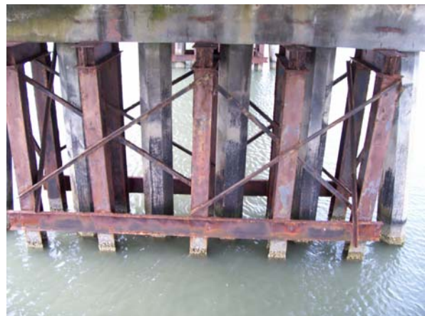
Bent 117: south elevation
