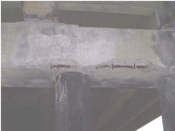
Bent 6, bent cap: north face, SP & ER
