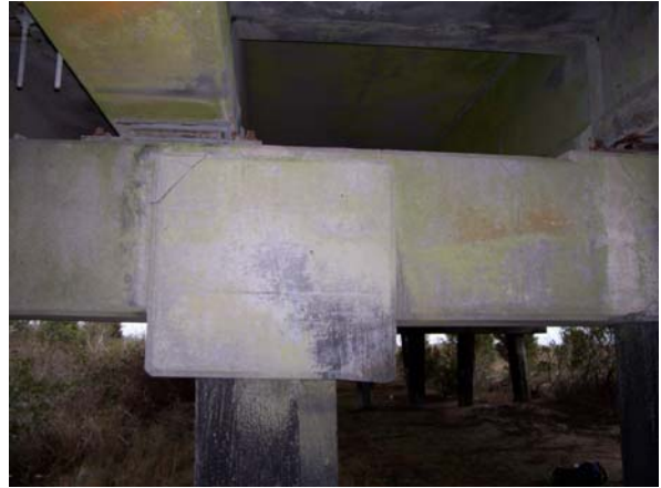
Bent 4, bent cap: North elevation
