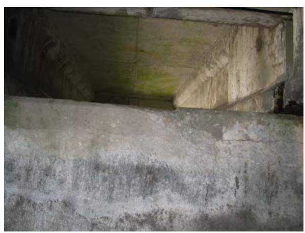
Bent 201: south elevation
