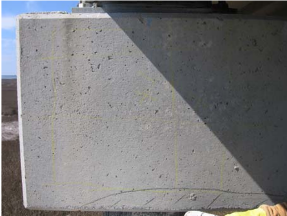
Bent 88, bent cap: south side
