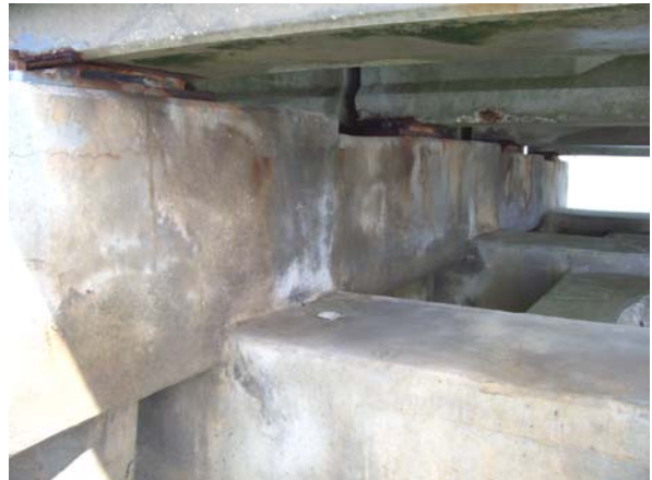
Bent 178: South elevation
