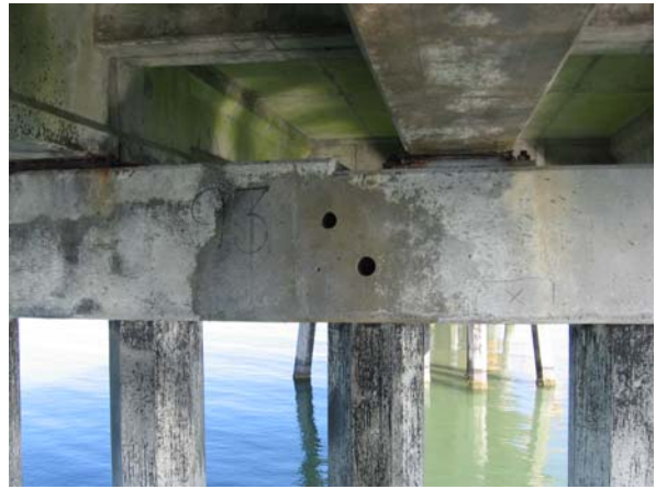
Bent 93, Bent cap: south face
