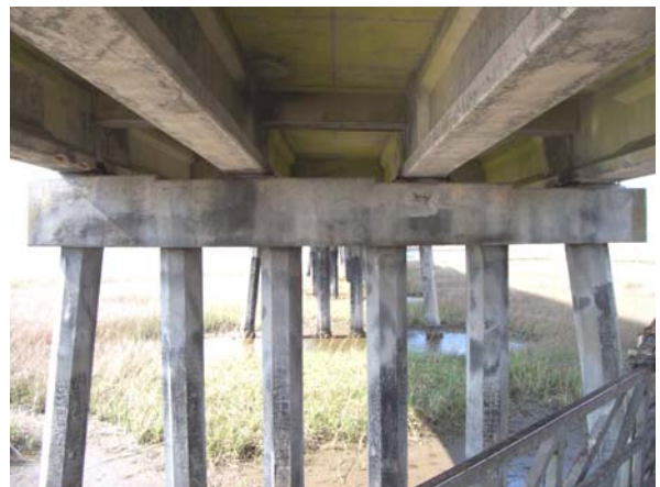
Bent 75: south elevation
