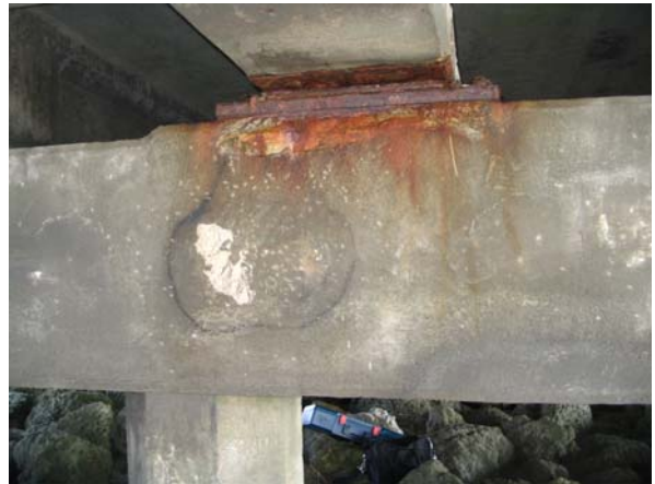
Bent 201: north elevation
