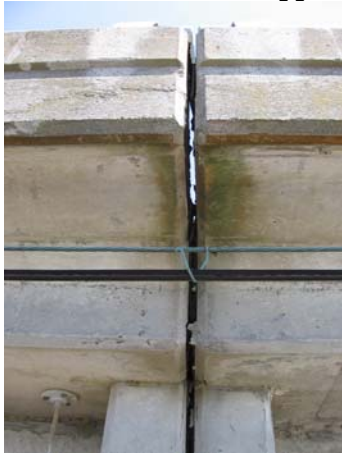
Bent 88: Girder ends and bearing, west side
