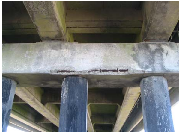
Bent 7; South Face
