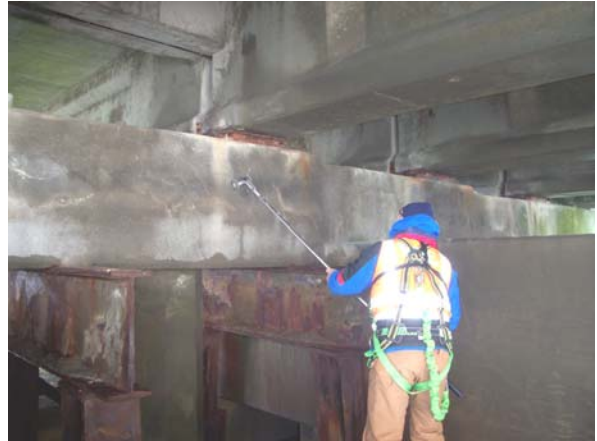
Bent 190: south elevation
