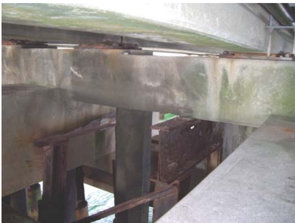
Bent 190: south elevation
