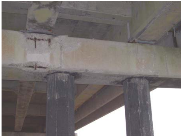
Bent 19: large SP
