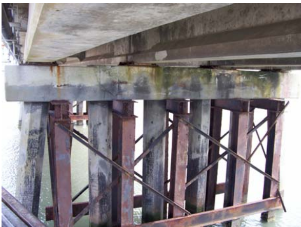
Bent 117: north elevation
