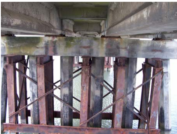
Bent 117: south elevation
