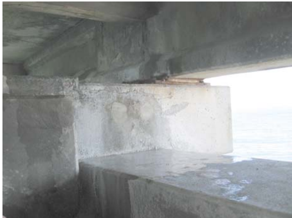
Bent 164, Bent cap: south face
