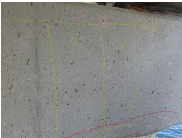
Bent 102, bent cap: south face, east end
