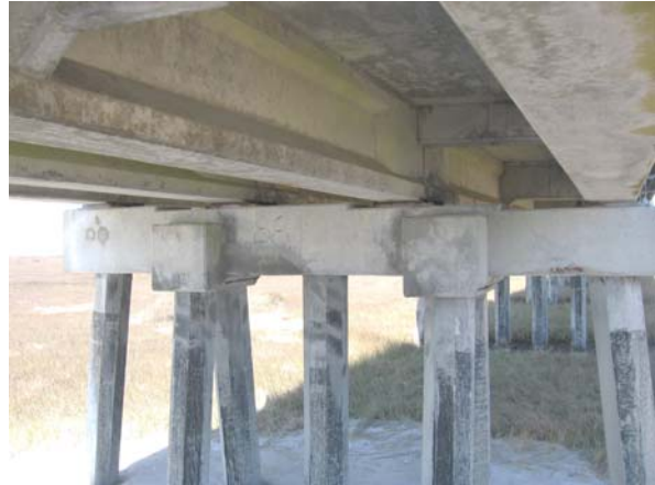
Bent 88: Bent cap, south elevation
