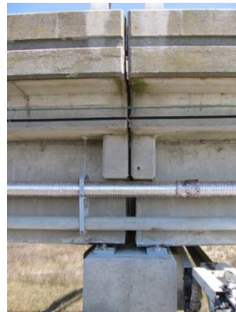
Bent 88: Girder ends and bearing, west side
