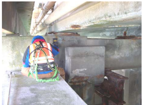
Bent 187: south elevation
