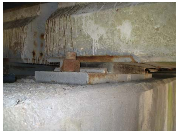
Bent 7; West side of Girder 4
