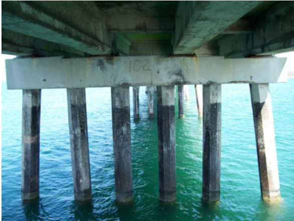
Bent 102: south elevation
