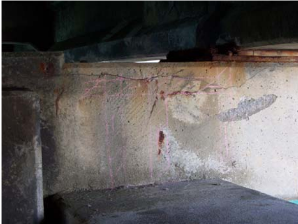
Bent 167: South Face
