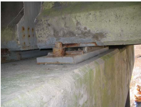
Bent 7; West side of Girder 2
