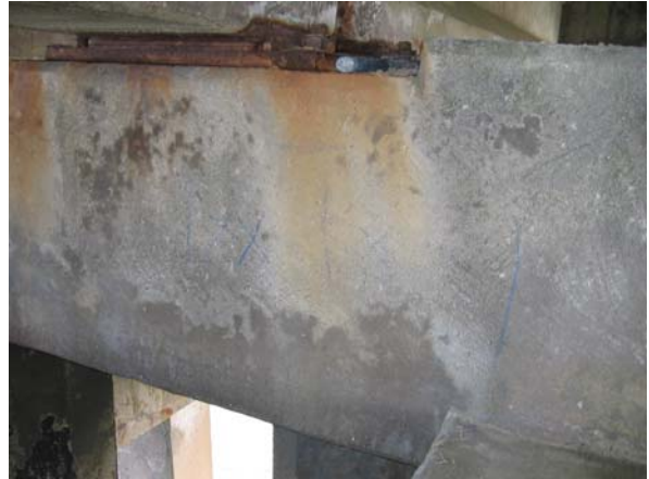
Bent 176: bent cap, north face
