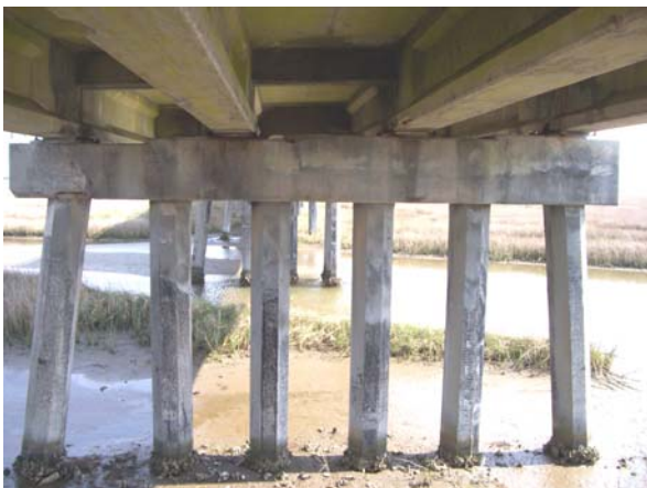
Bent 75: north elevation
