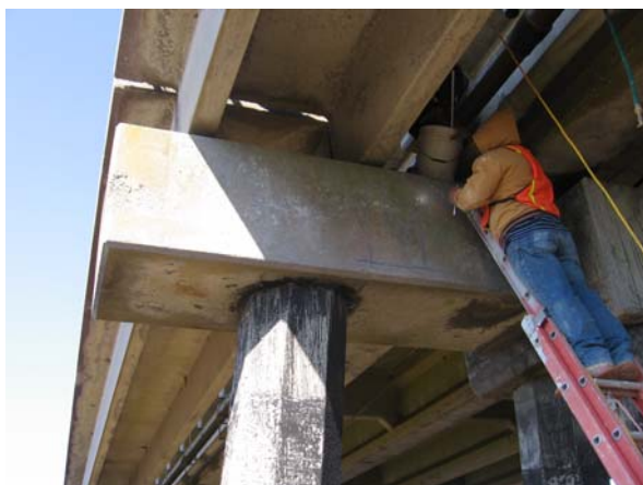
Bent 12: Bent cap, south face
