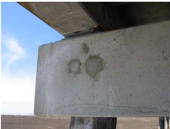
Bent 88: Bent cap, south elevation, west end
