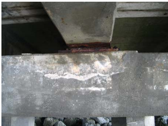
Bent 201: north elevation
