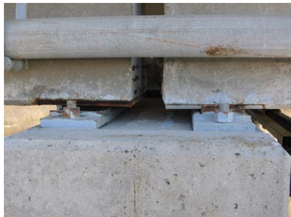
Bent 88: Girder ends and bearing, west side
