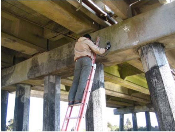
Bent 7; Top of bent cap
