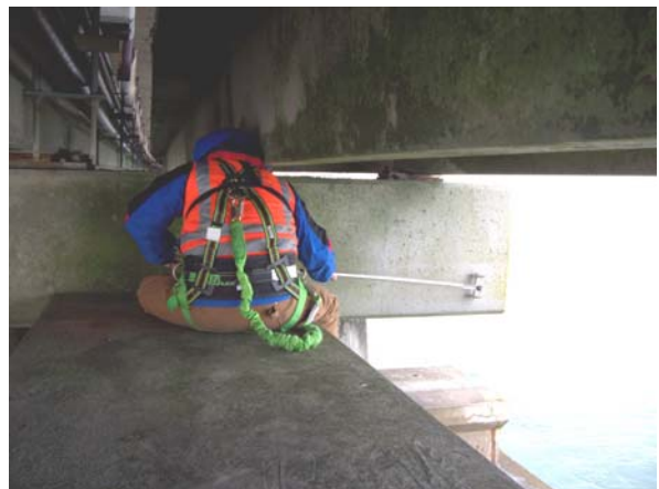
Bent 190: south elevation
