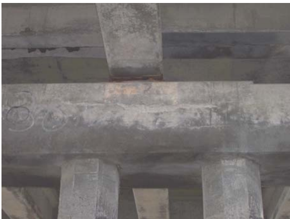
Bent 38: large SP @ bearing
