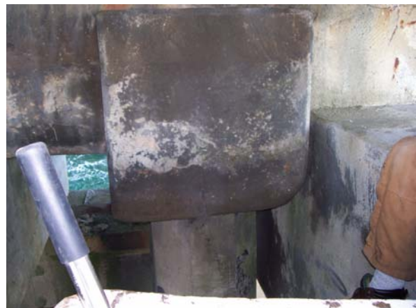
Bent 167: south elevation
