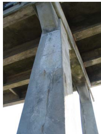
Bent 160, East external side
