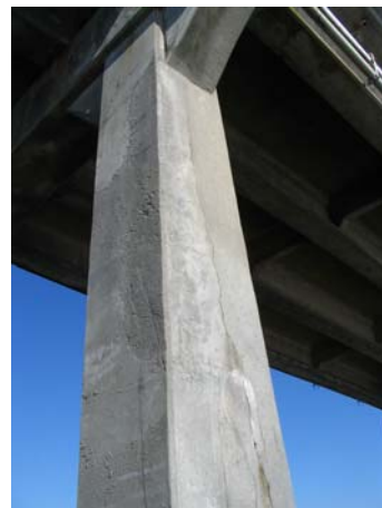
Bent 160, west column: north elev
