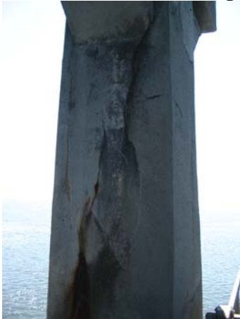
Bent 163, west interior side
