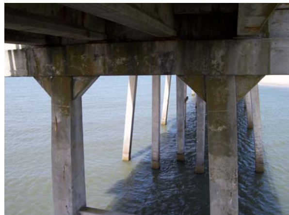
Bent 129, South elevation; bent cap
