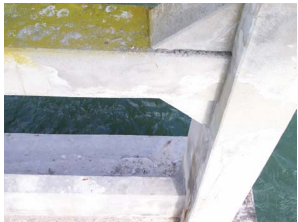
Bent 149, pile cap: south elev
