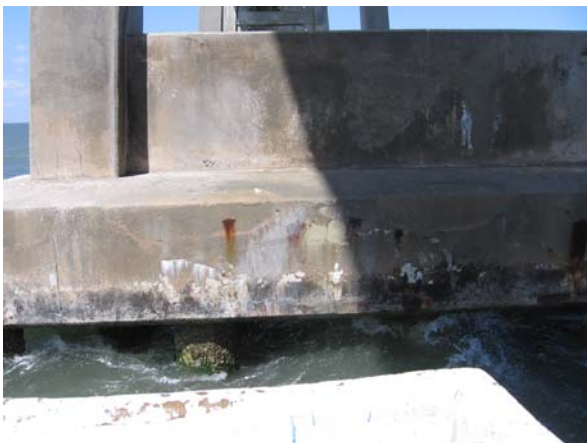
Bent 154, Pile cap: south face, west end
