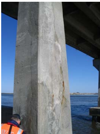
Bent 160, west column: north elev
