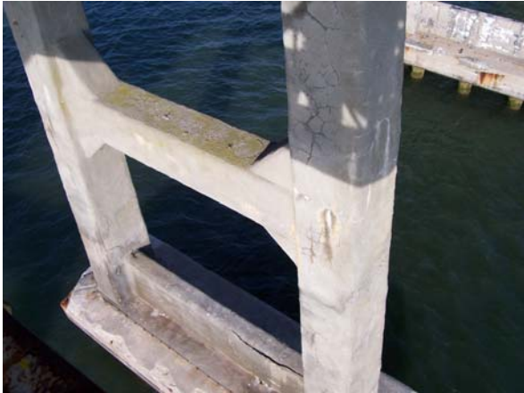
Bent 135, South elevation; pile cap & middle
