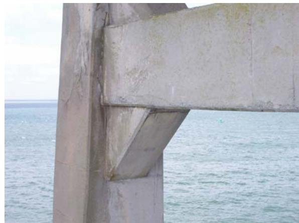
Bent 149, bent columns: south elev
