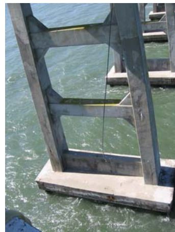
Bent 150, south elevation
