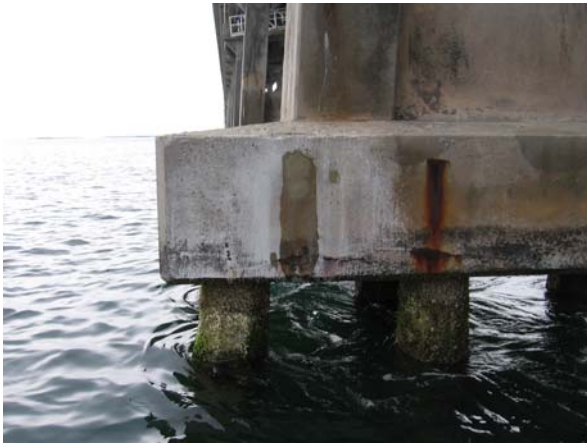
Bent 163, Pile cap: south face, west end
