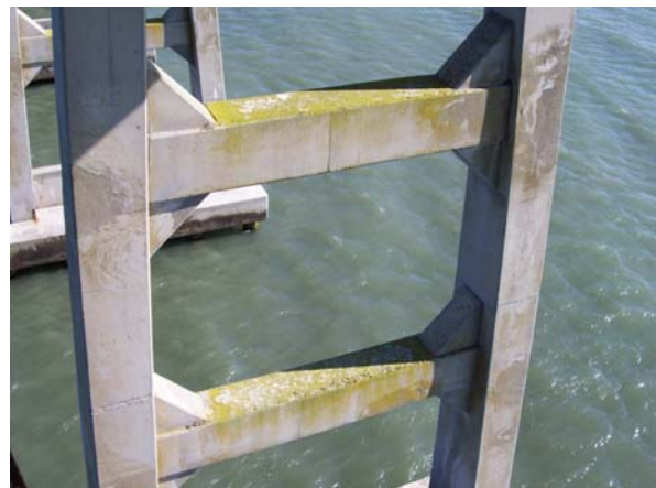
Bent 140, North elev; middle columns of bent
