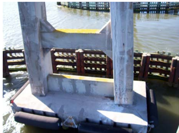
Bent 145, South elev: pile cap & lower cross
