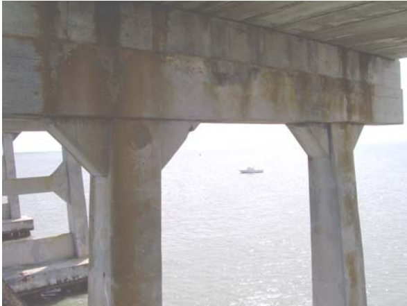
Bent 129, North elevation; bent cap
