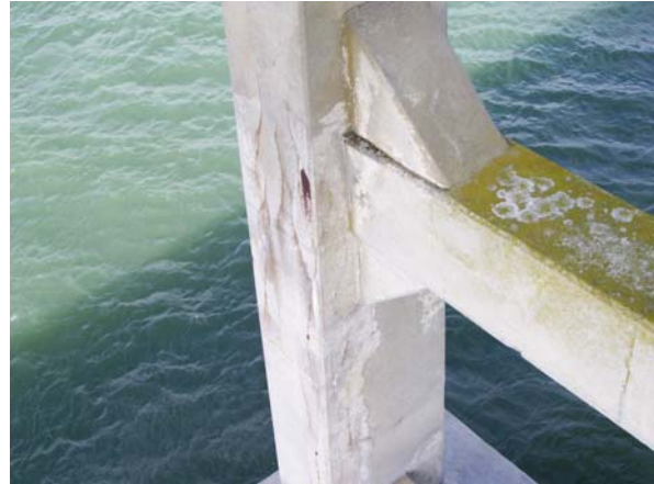
Bent 149, bent columns: south elev
