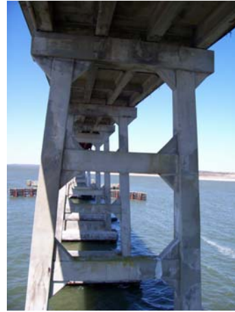
Bent 149, bent cap and upper columns: south
