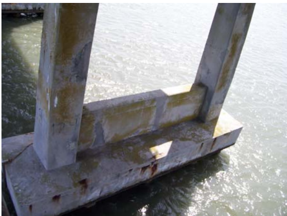
Bent 129, North elevation; pile cap
