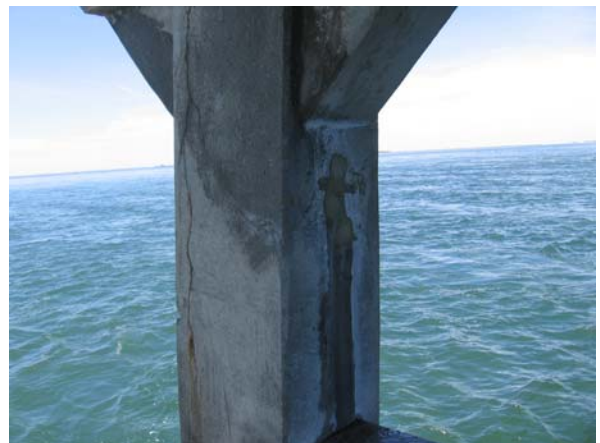
Bent 164, West column: west interior side
