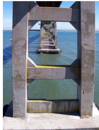
Bent 145, North elev: lower 3/4 of bent
