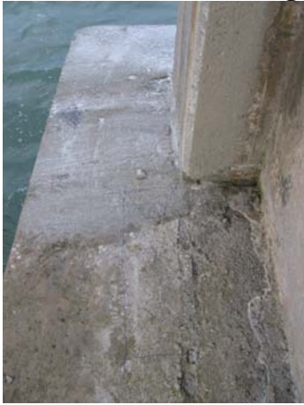
Bent 160, Pile cap: top face, NE corner
