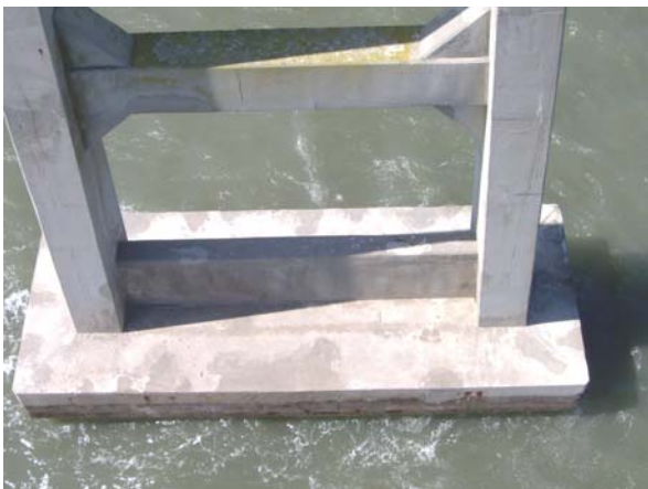
Bent 140, South elev; pile cap & lower beams
