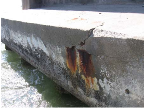
Bent 150, pile cap: south elev
