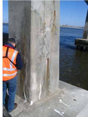
Bent 160, west column: north elev
