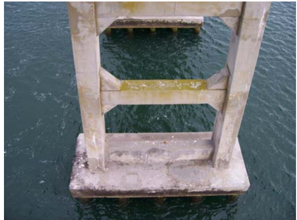
Bent 150, lower 1/2: north elev
