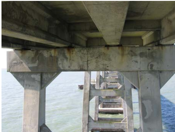
Bent 150, south elevation
