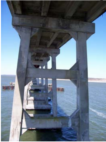
Bent 149, bent cap and upper columns: south
