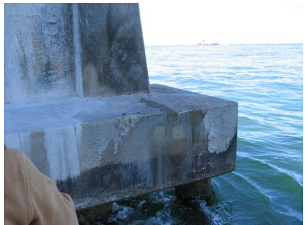
Bent 164, Pile cap: south face, east end
