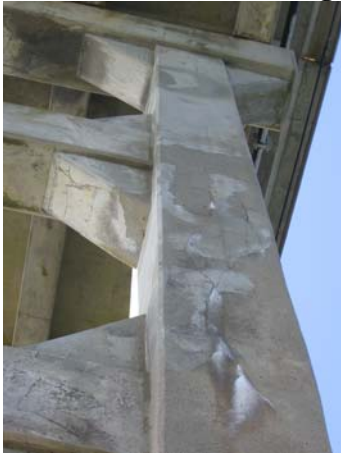
Bent 150, east column: south elev
