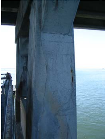
Bent 163, east exterior side
