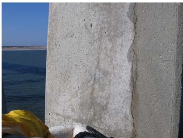
Bent 150, West column: west exterior side, mid
