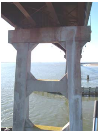
Bent 145, South elev: upper 1/2 of bent
