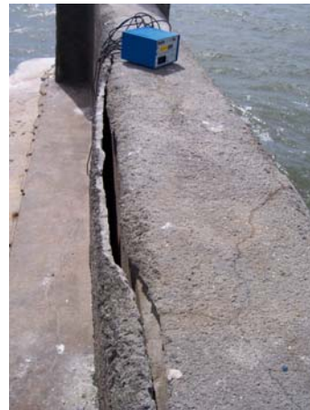
Bent 135, South elev; lower beam DL close-up
