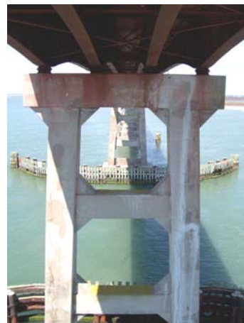
Bent 145, South elev: upper 3/4 of bent
