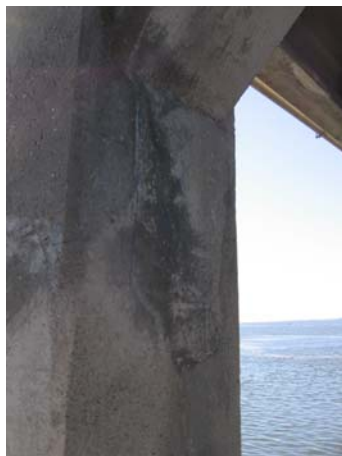
Bent 164, West column: west interior side
