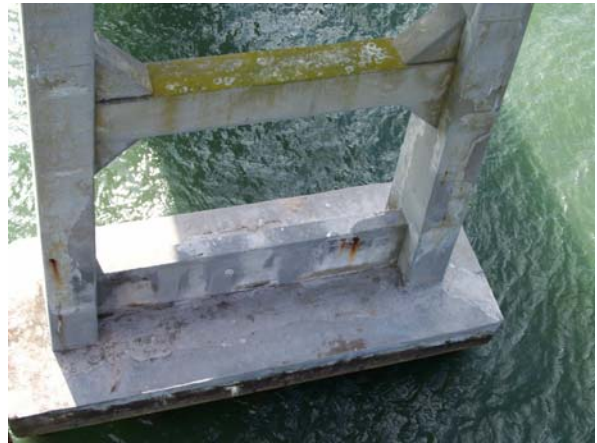
Bent 149, pile cap: north elevation
