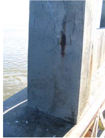
Bent 160, East external side
