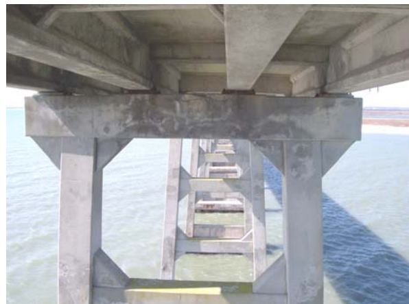
Bent 140, South elev; bent cap & upper columns
