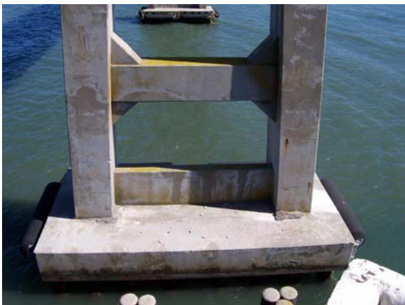
Bent 145, North elev: lower 1/2 of bent
