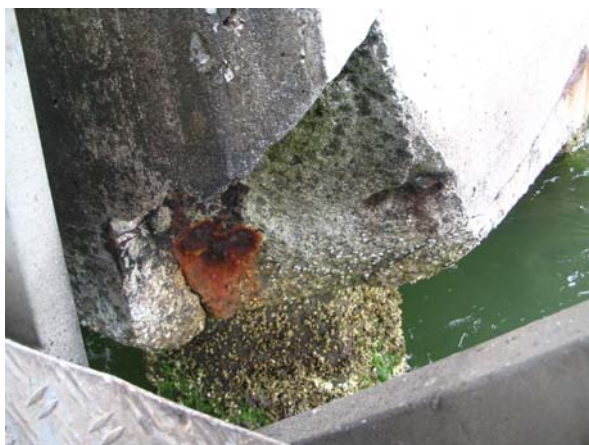
Bent 164, west exterior side
