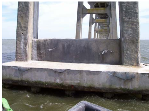
Bent 135, South elevation; pile cap & lower
