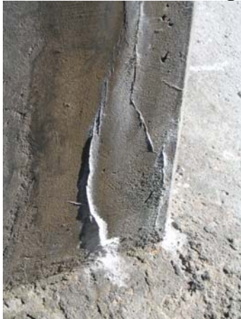
Bent 160, west column: north elev
