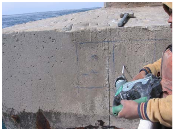
Bent 163, Pile cap: south face, west end
