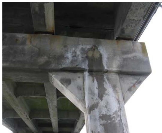
Bent 163, Bent cap: south face, east end
