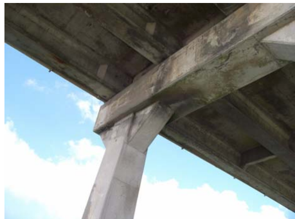
Bent 149, bent cap: south elev
