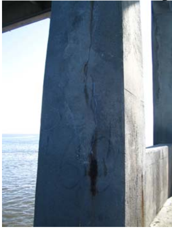
Bent 160, East external side
