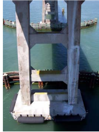
Bent 145, South elev: lower 3/4 of bent
