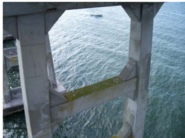
Bent 149, columns: north elevation
