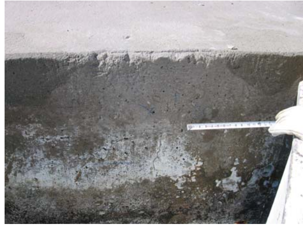
Bent 150, Pile cap: south face, east end
