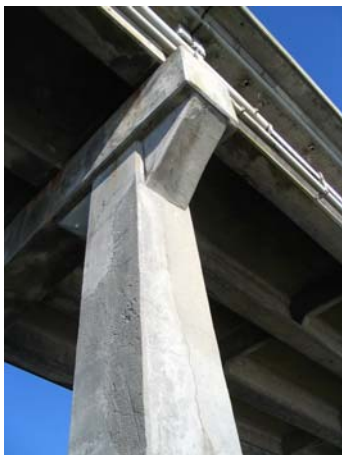
Bent 160, west column: north elev
