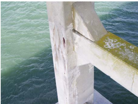
Bent 149, bent columns: south elev
