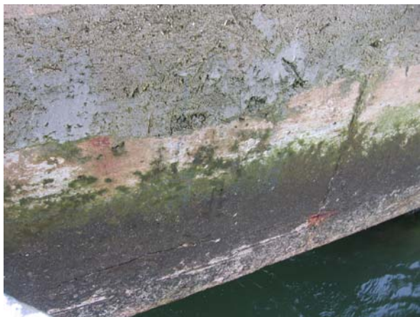
Bent 160, Pile cap: north face, west end
