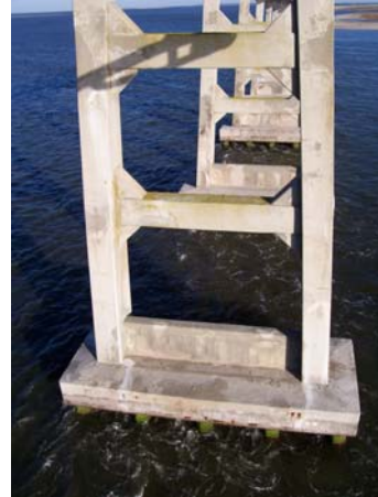
Bent 140, South elev; lower 3/4 of bent
