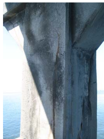
Bent 163, west interior side
