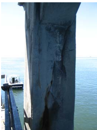
Bent 163, west interior side
