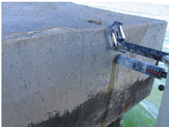
Bent 164, Pile cap: south face, east end
