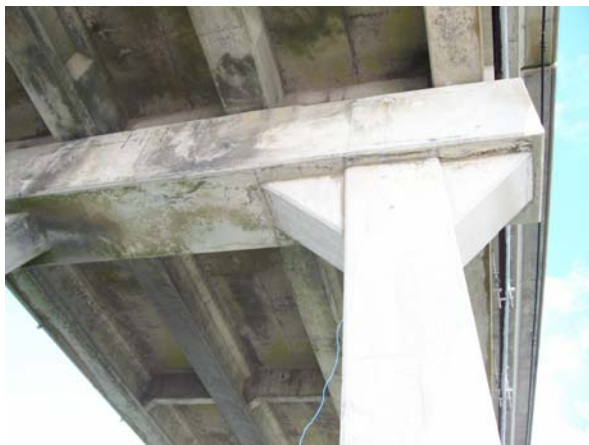
Bent 149, bent cap: south elev
