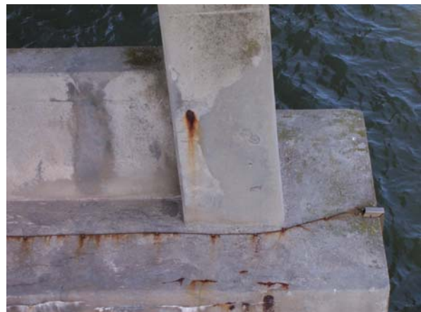
Bent 129, South elevation; pile cap East end
