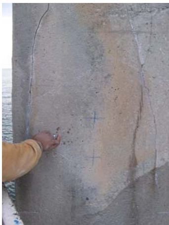
Bent 163, East column: east exterior side
