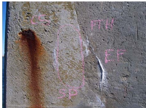
Bent 149, east column: CS EF & SP
