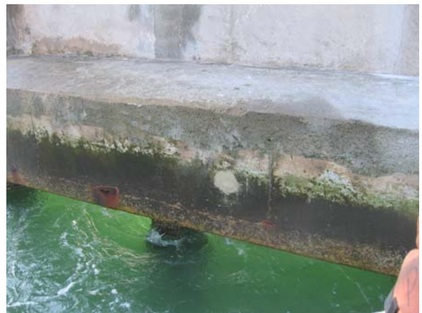
Bent 160, Pile cap: north face, west end
