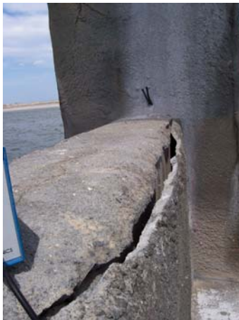
Bent 135, South elev; lower beam DL close-up
