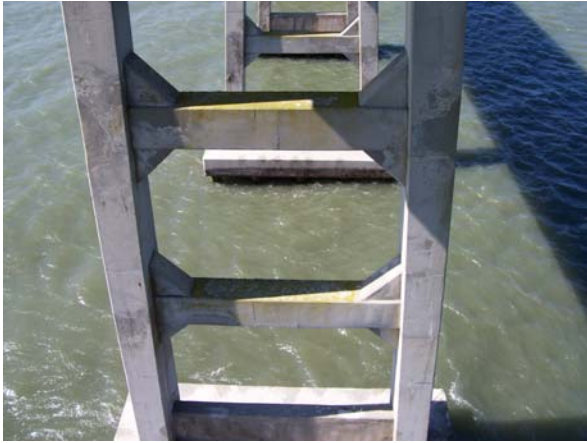
Bent 140, South elev; columns & cross beams
