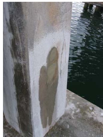
Bent 163, East column: east exterior side
