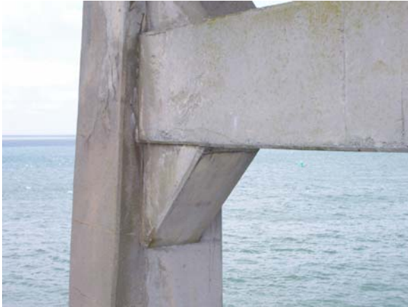
Bent 149, bent columns: south elev
