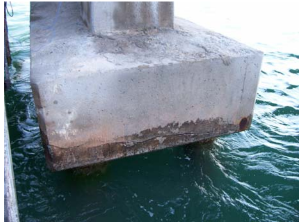
Bent 161, pile cap; west elev
