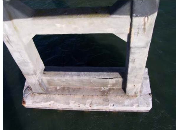
Bent 135, South elevation; pile cap shot from
