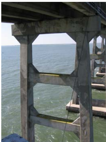
Bent 150, south elevation
