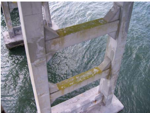
Bent 149, columns: north elevation
