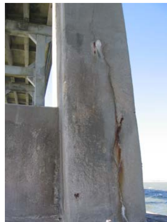
Bent 150, east column: south elev
