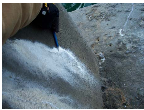
Bent 161, CS CR EF on west exterior side
