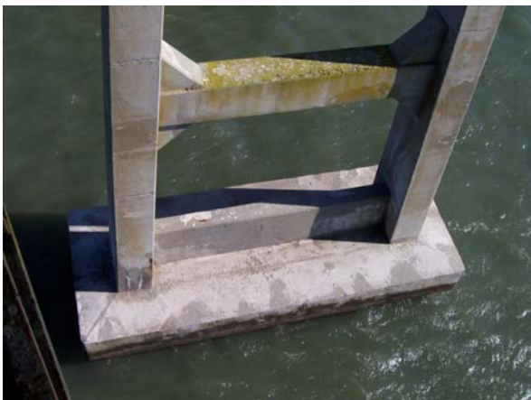
Bent 140, North elev; pile cap & lower beams
