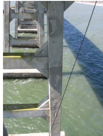
Bent 150, south elevation
