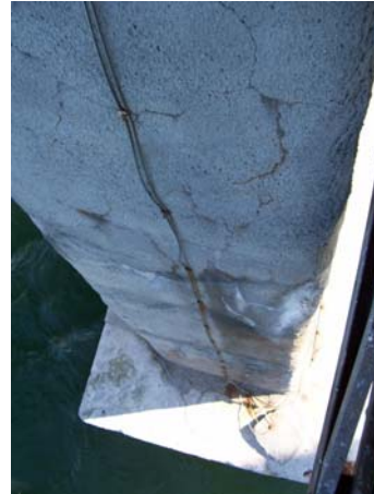
Bent 135, South elev; cathodic protection, shot
