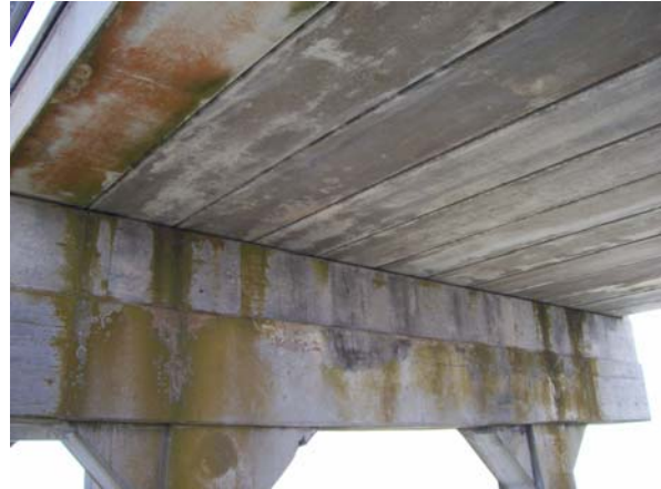
Bent 129, North elevation; bent cap
