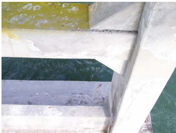
Bent 149, pile cap: south elev
