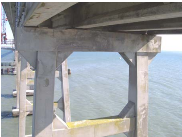
Bent 140, North elev; bent cap & upper columns
