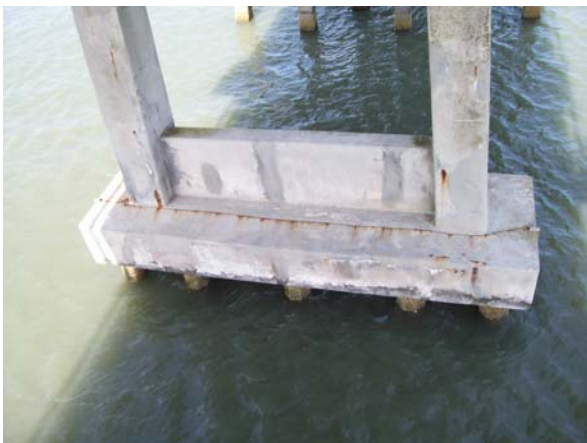
Bent 129, South elevation; pile cap
