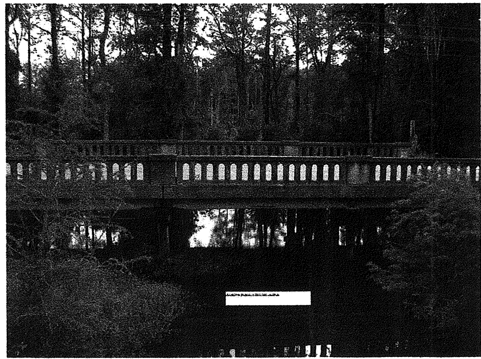
View of Interior bents 1 and 2 looking North
