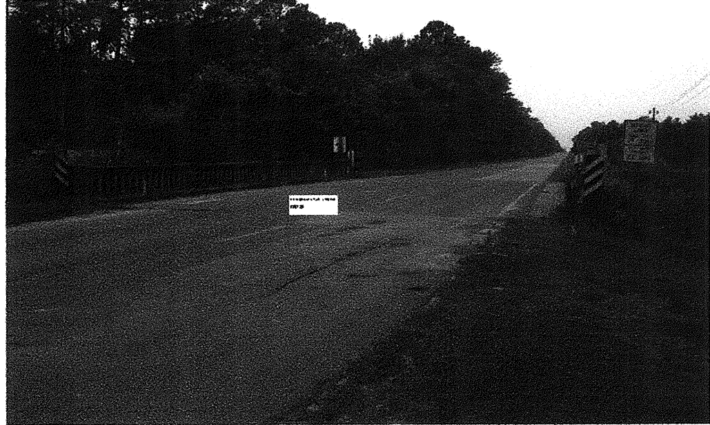
View along "B" borings from End Bent 2 towards End Bent 1
