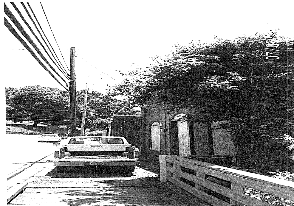
Photograph 6 – View Along Right Side of Existing Bridge Looking Upstation
