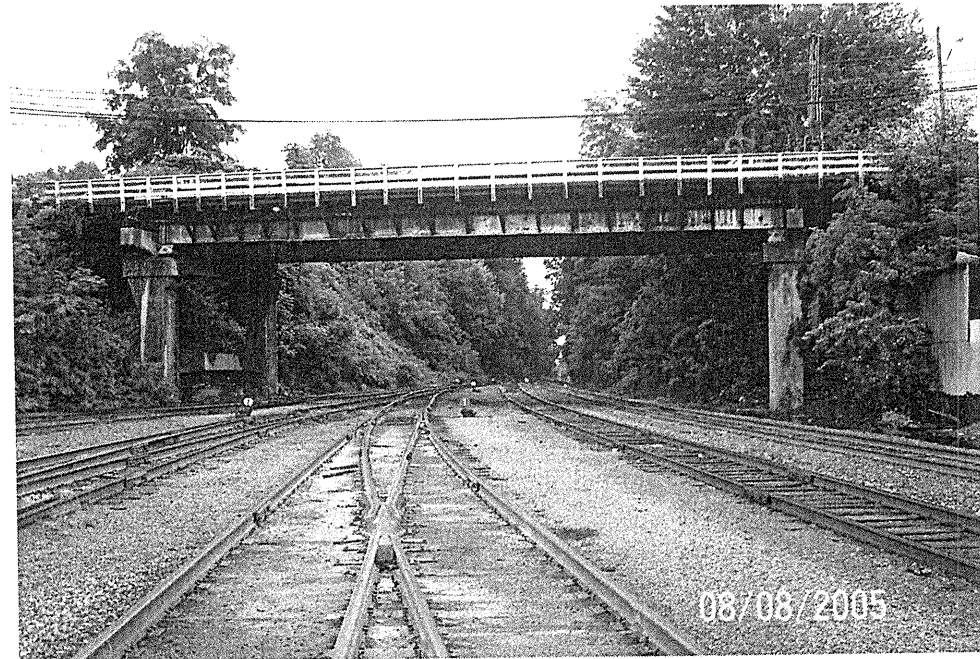
Photograph 10 – View of Existing Bridge Looking East
