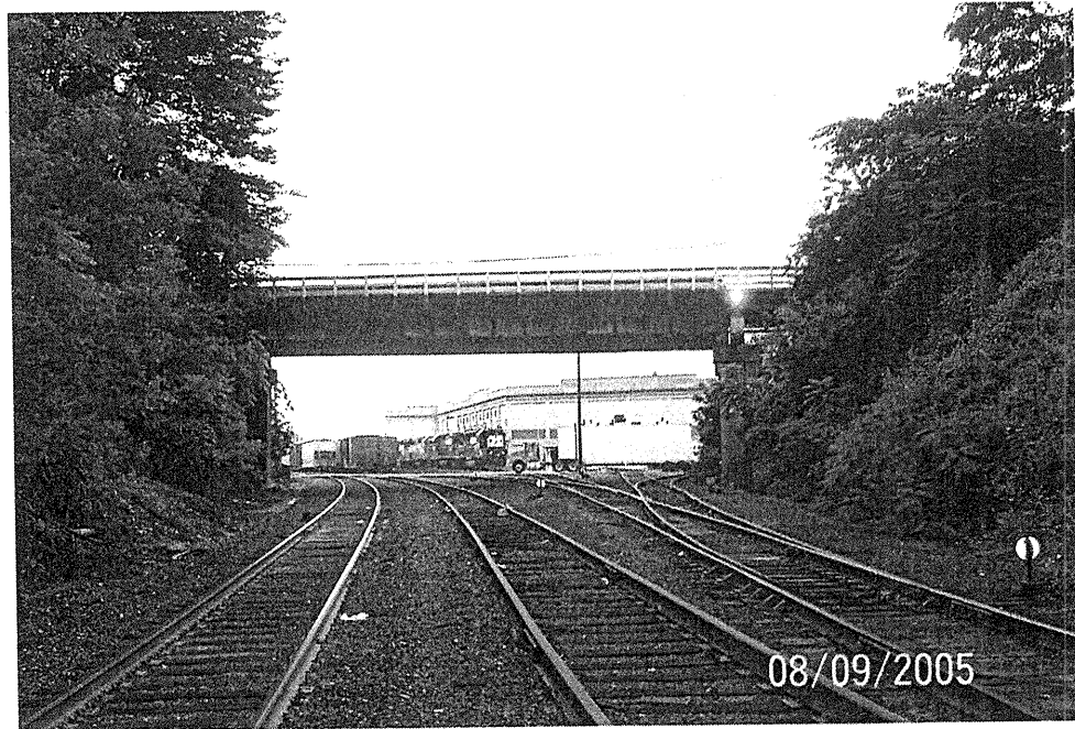
Photograph 9 – View of Existing Bridge Looking West
