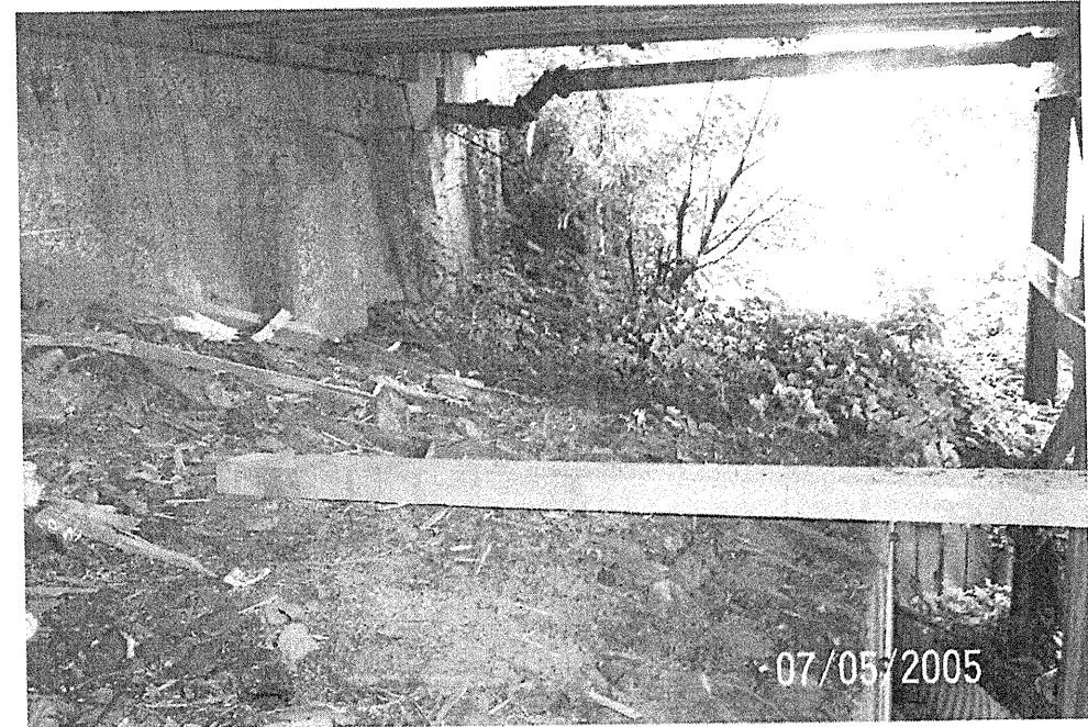
Photograph 7 – View of Existing End Bent-2 Abutment
