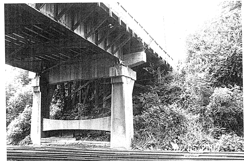
Photograph 8 – View of Existing End Bent-1
