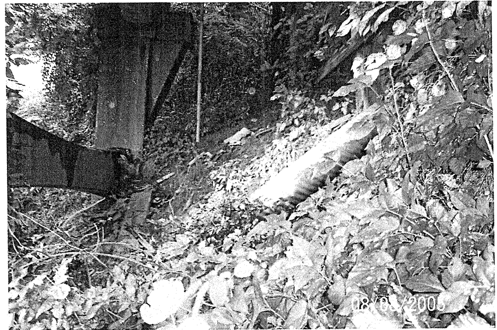
Photograph 4 – View Along Proposed End Bent-2 Looking Right to Left
