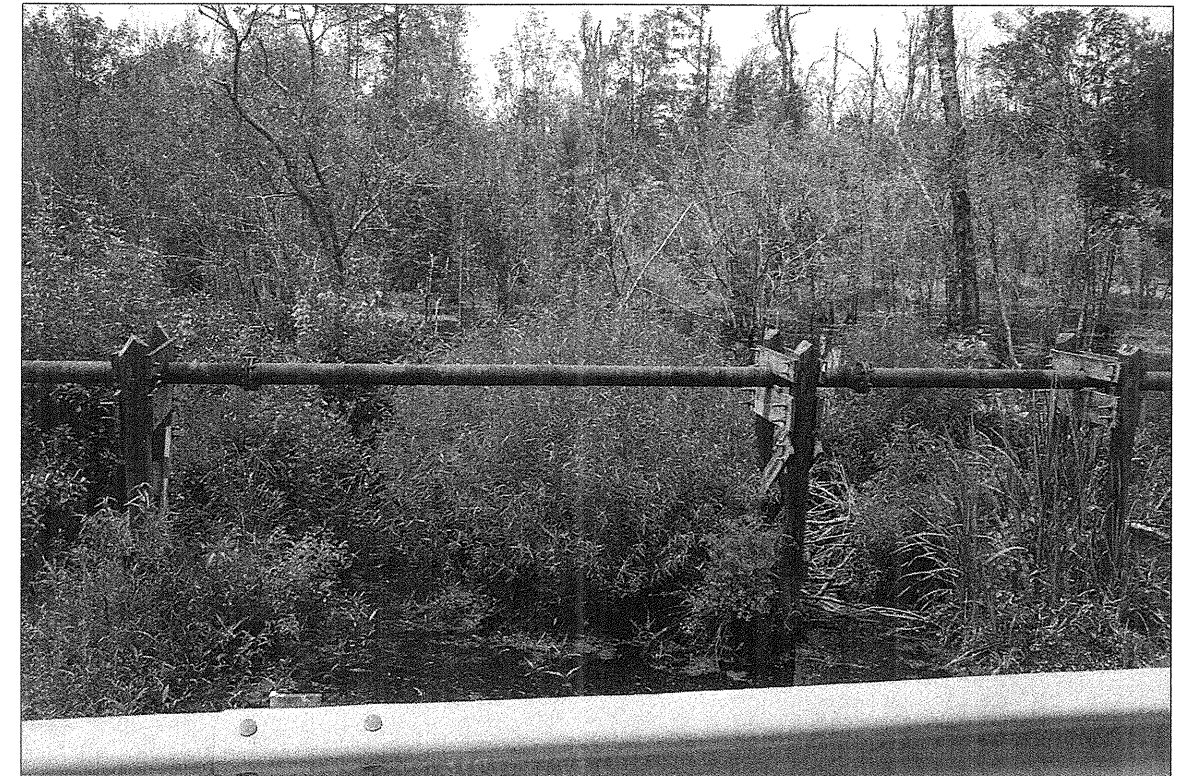
BENT 1 FACING UPSTREAM TO THE NORTHWEST
