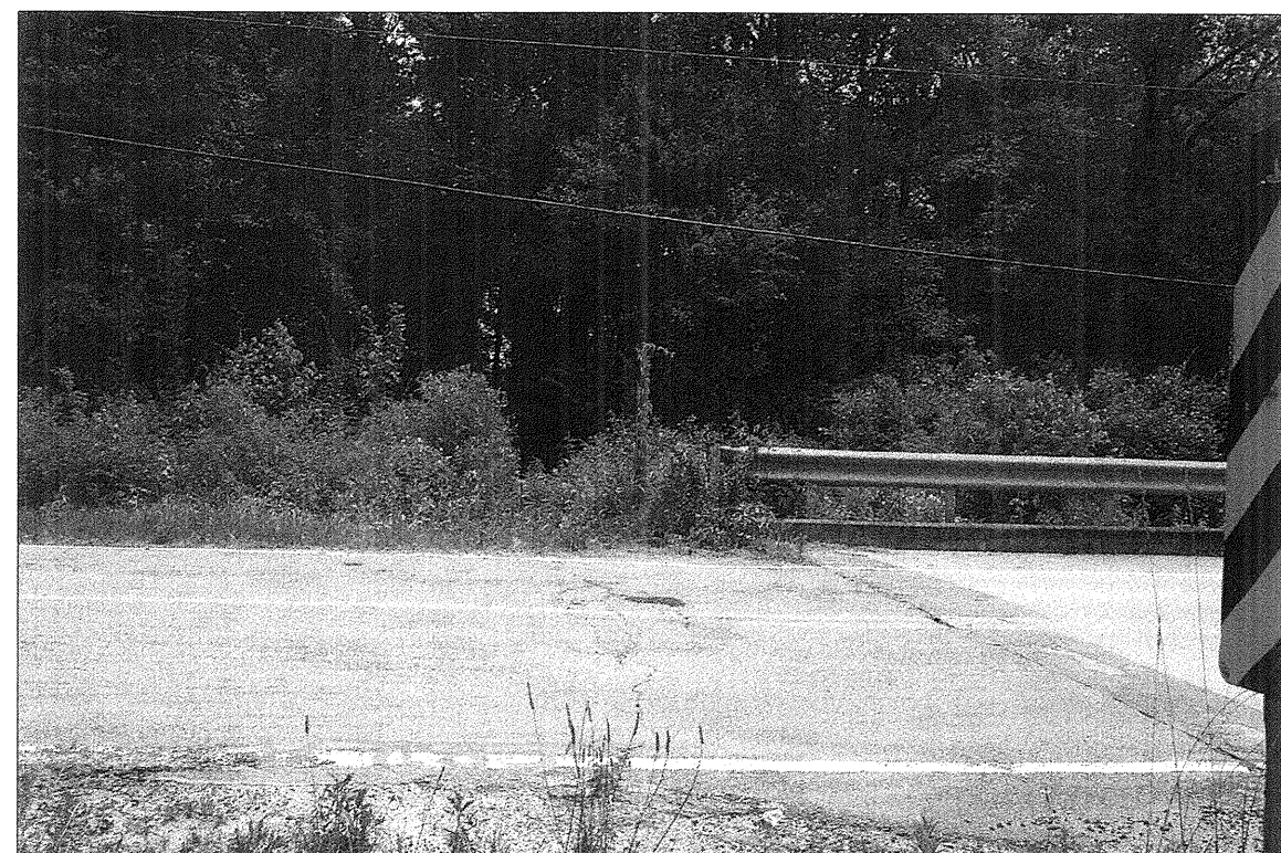
SECTION ACROSS END BENT 2 FACING SOUTHEAST EB2A IN FOREGROUND
