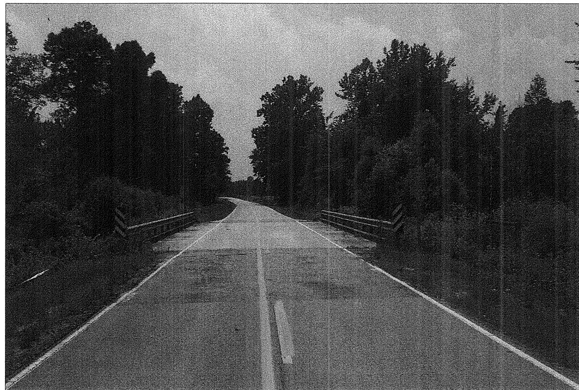
CENTERLINE OF -L- END BENT 2 IN FOREGROUND FACING SOUTHWEST
