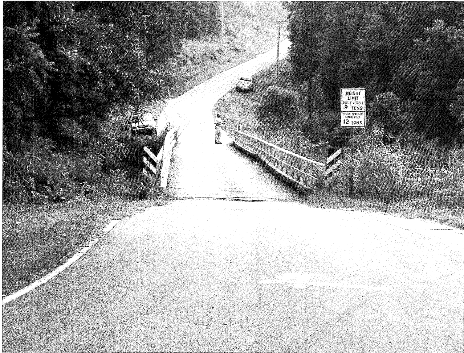
EXISTING BRIDGE LINE AHEAD
