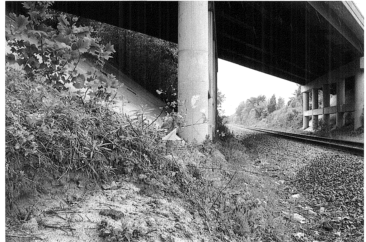
Photograph 7: View Along Bent-2 From Left to Right
