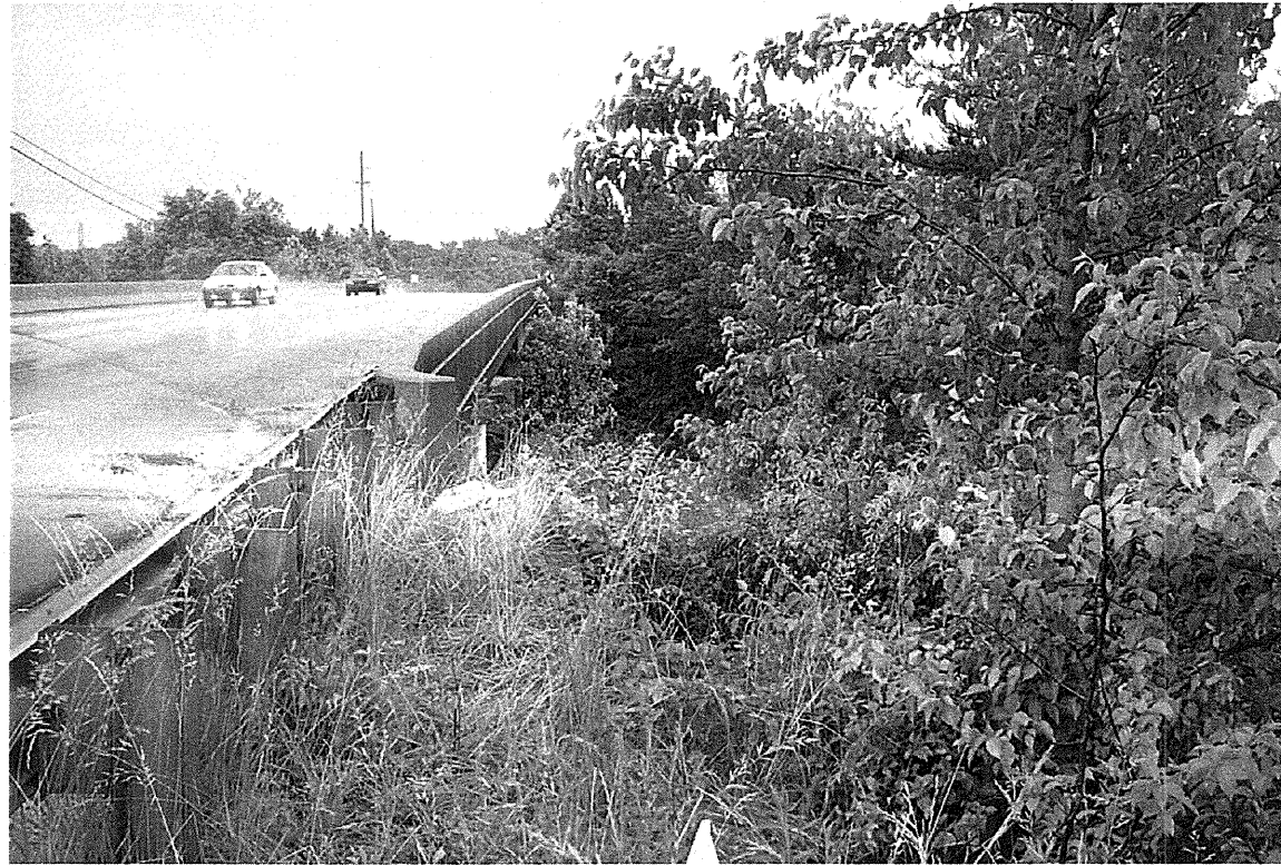
Photograph 1: View 9m Right of -L- from North of End Bent-1
