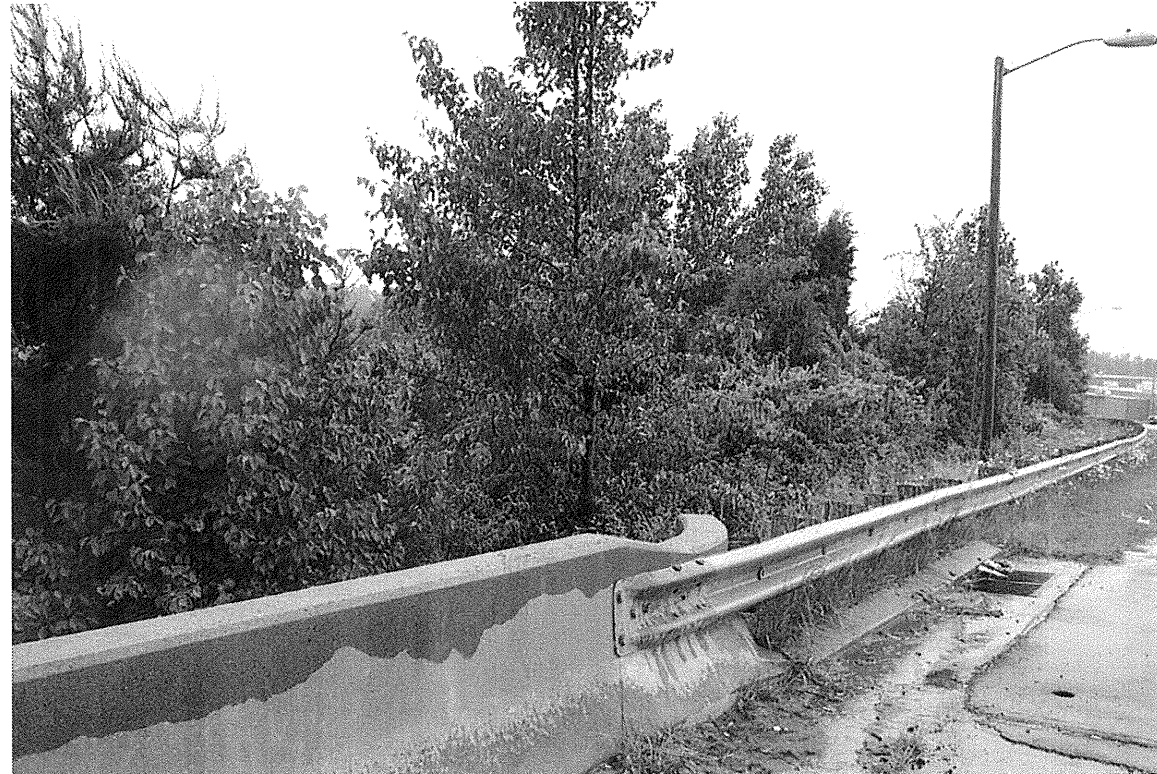
Photograph 5: View Along End Bent-1 From Edge of Road Towards EB1-B Plan
