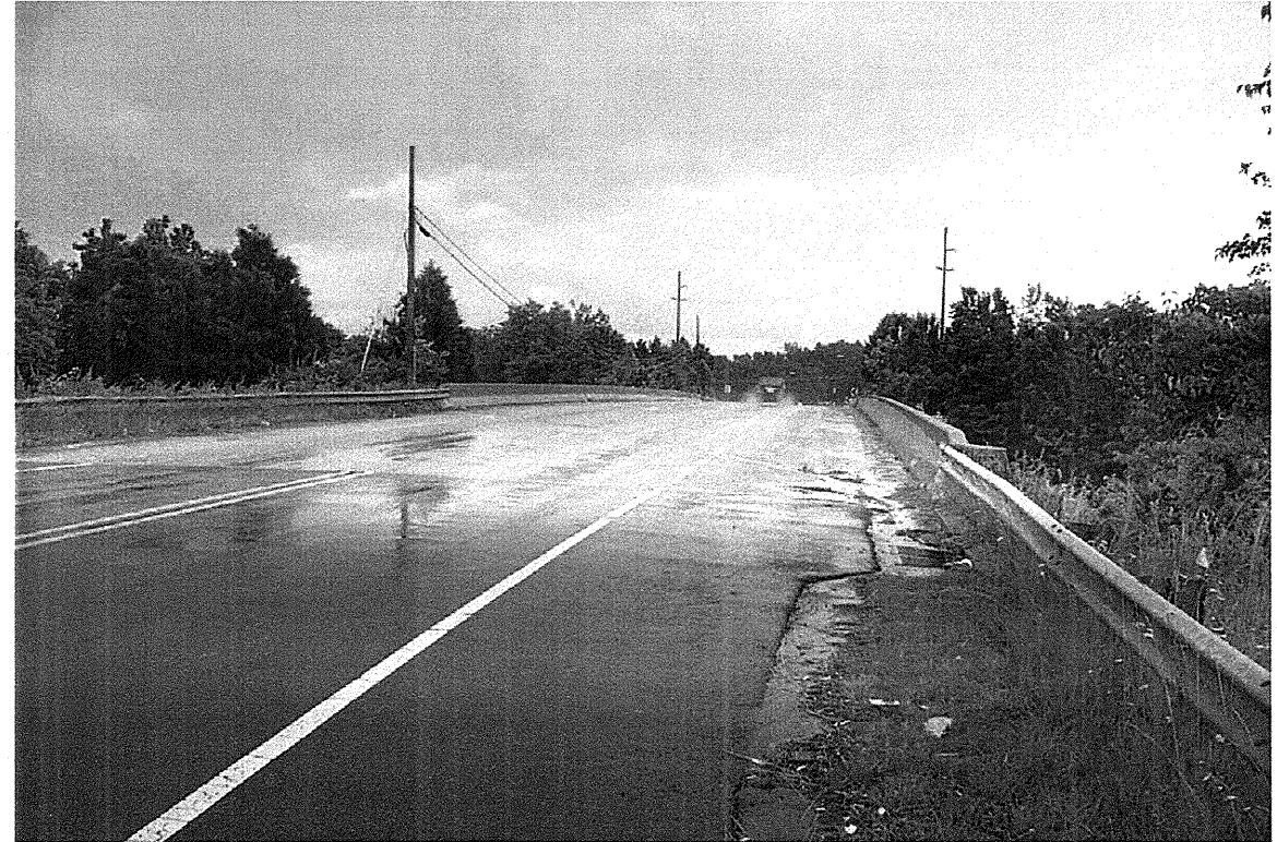
Photograph 11: View of Existing Bridge Looking South
