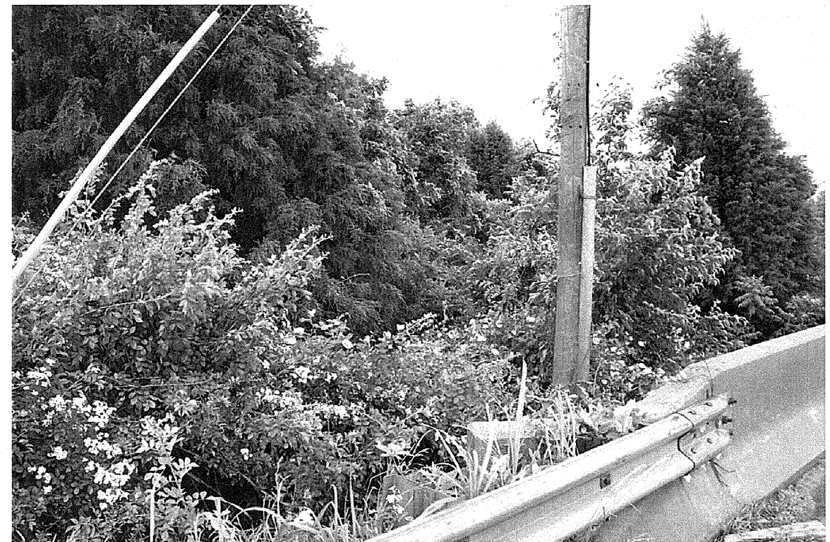
Photograph 4: View Along End Bent-1 From Edge of Road Toward EB1-A Plan
