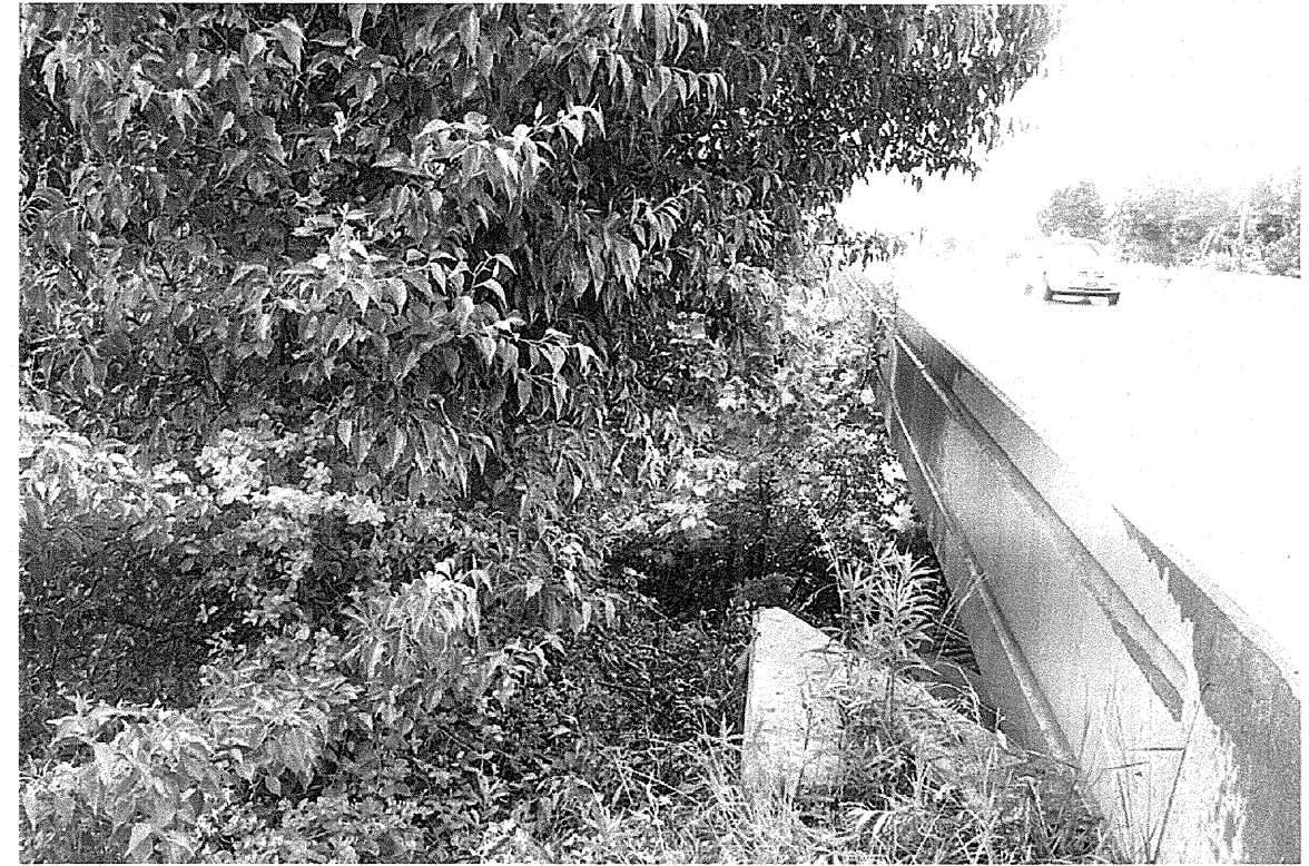
Photograph 3: View 9m Right of -L- From End Bent-2
