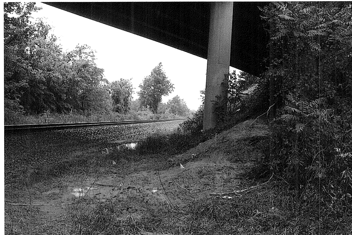
Photograph 6: View Along Bent-1 From Left to Right
