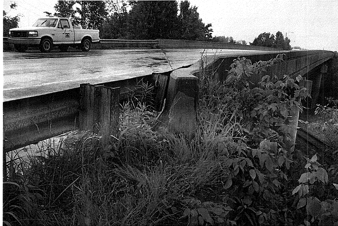
Photograph 9: View Along End Bent-2 From Left to Right
