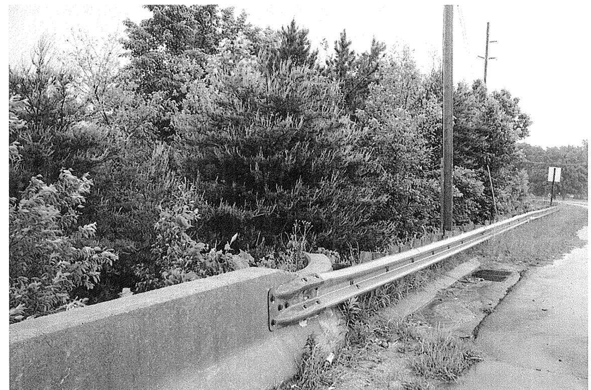
Photograph 8: View Along End Bent-2 From Edge of Road Toward EB2-A Plan
