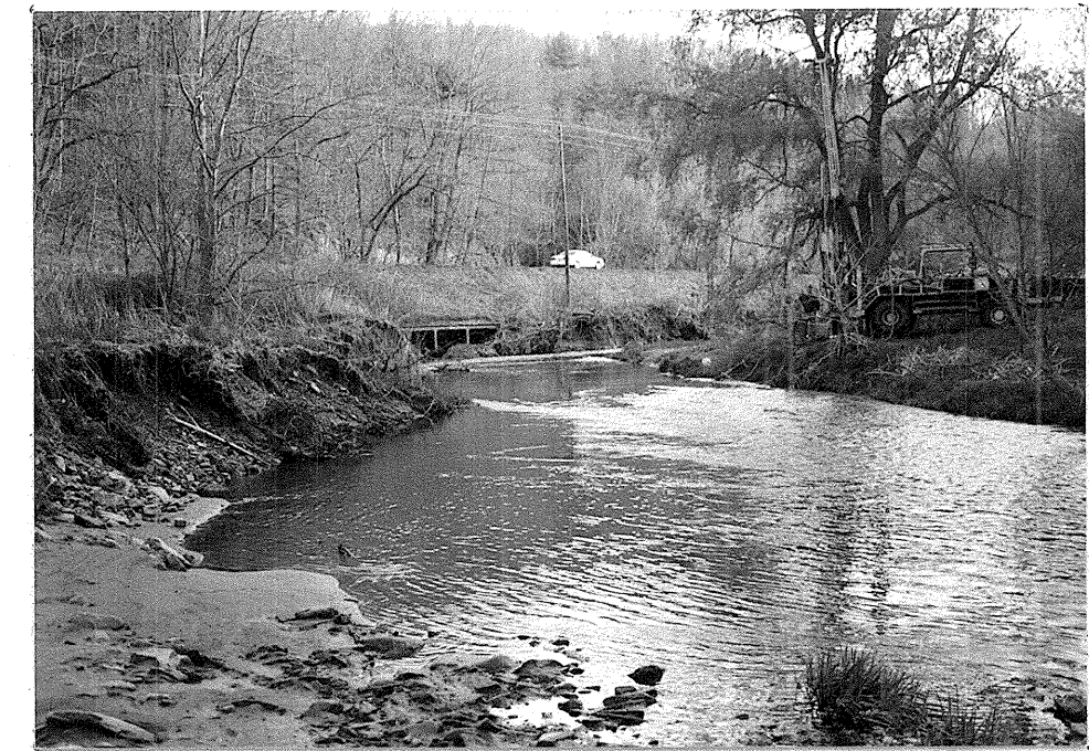
Figure 4. View looking upstream across -L-. Drilling on B1-A. Note fresh erosion on stream bank at B2 and at base of US 321 embankment.
