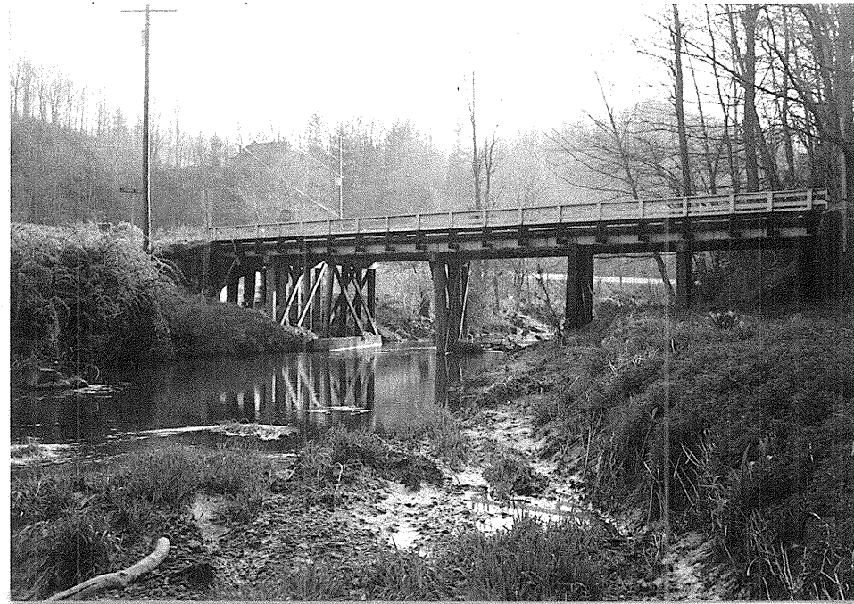
Figure 1. Bridge 316 on SR 1149. View looking upstream.
