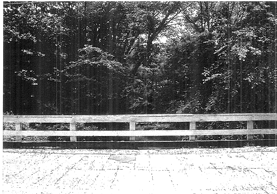
Looking Left to Right along Bent-1
