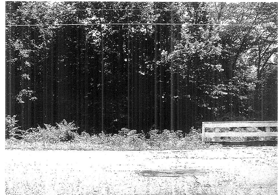
Looking Left to Right along End Bent-2
