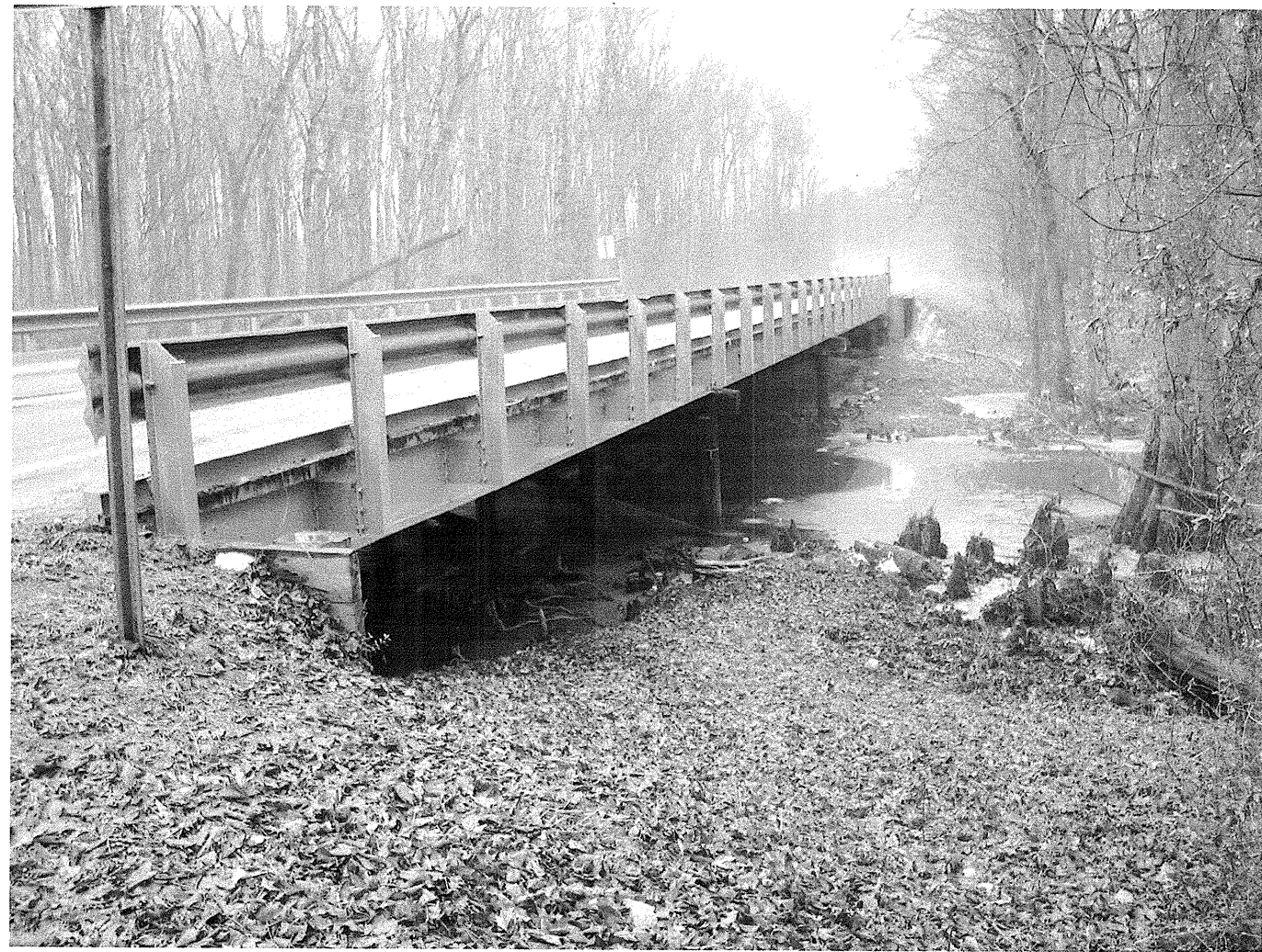
Looking east towards End Bent 2
