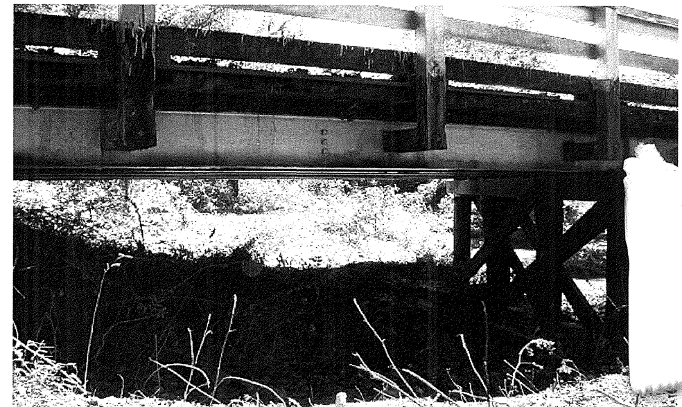
Looking Left to Right along Bent-2
