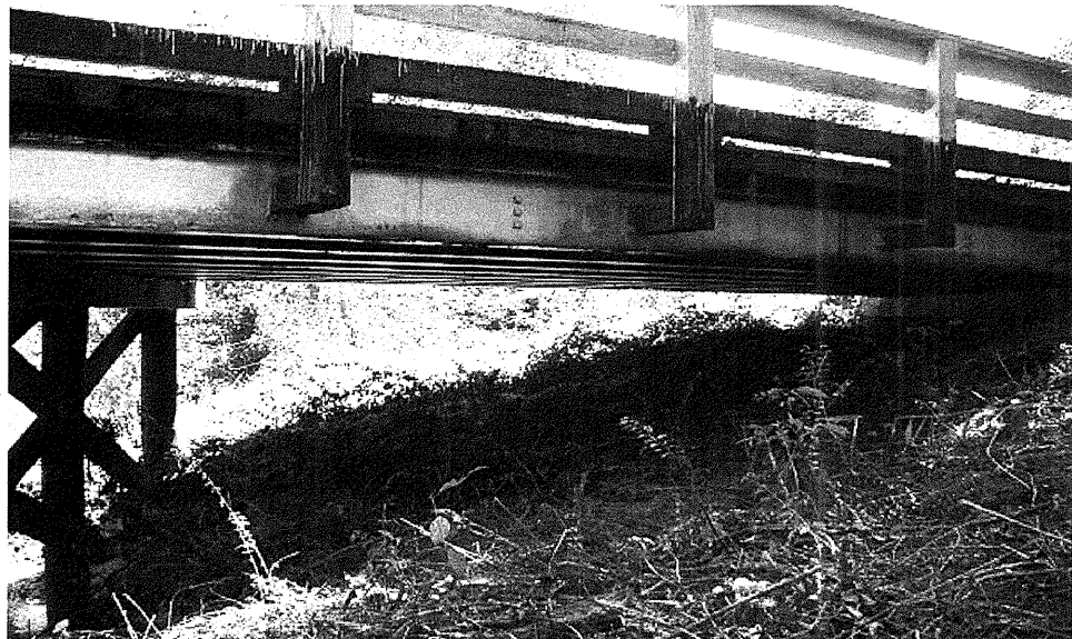
Looking Left to Right along Bent-1
