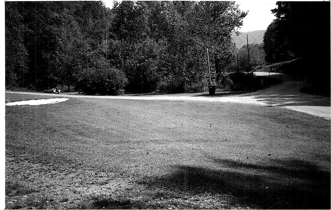
Fig. 3 Looking forward from a point near Centerline, Station 11+80
