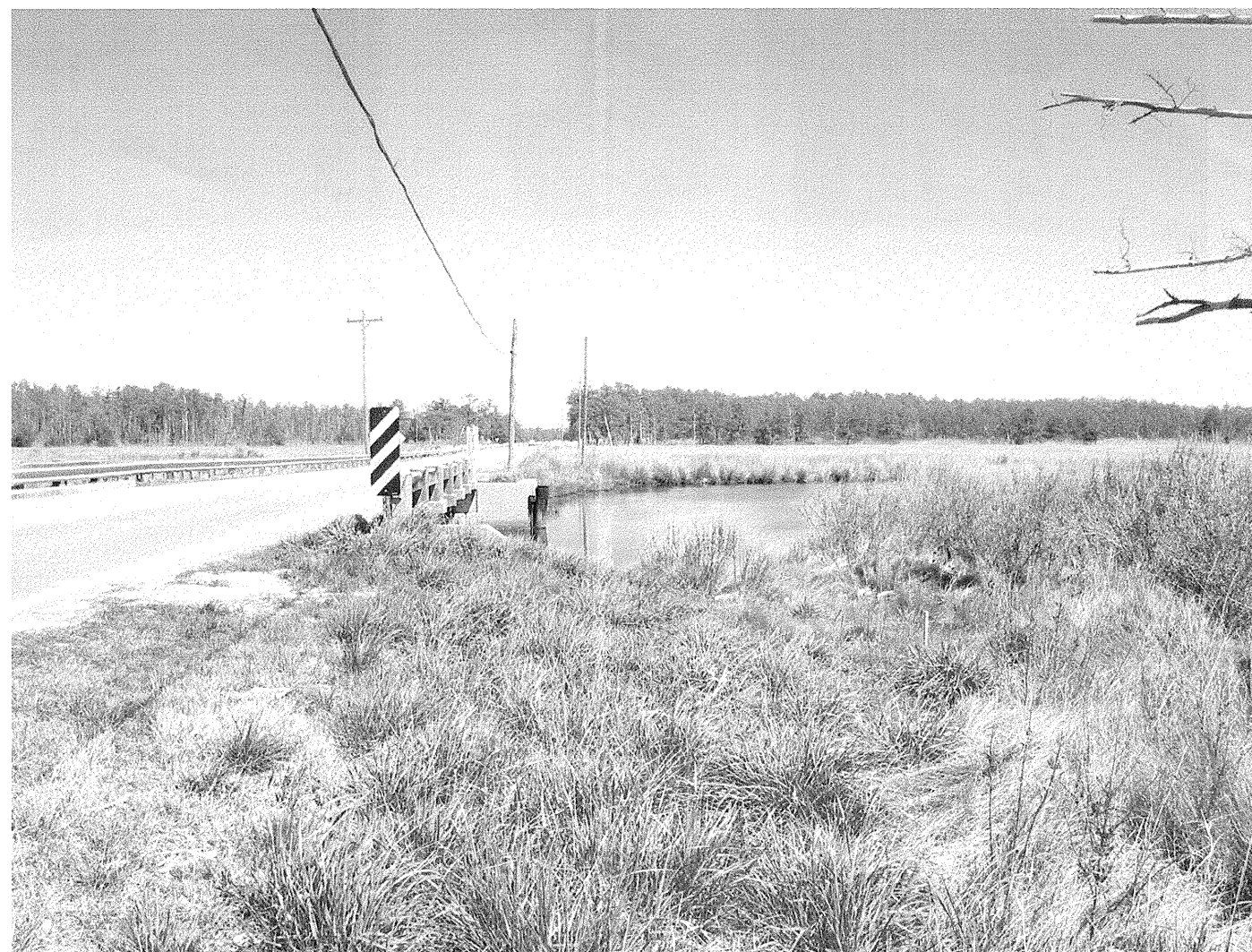
Looking north towards End Bent 2
