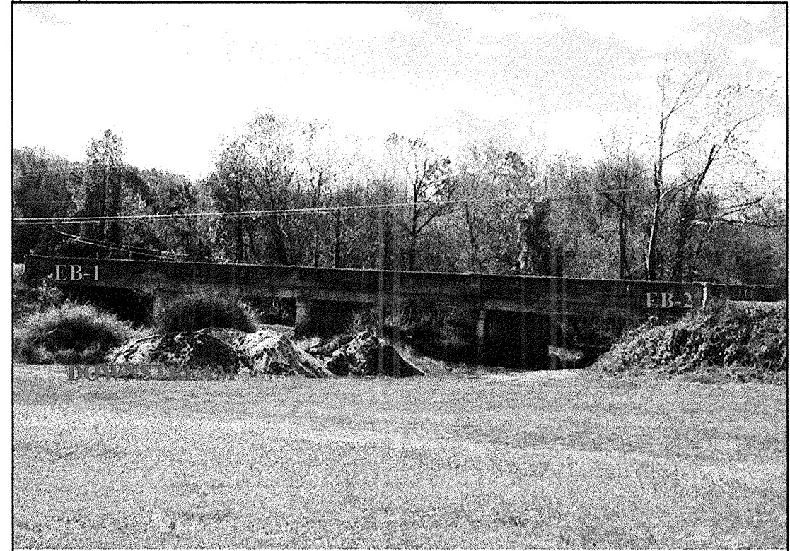
Looking at Bridge from Downstream.
