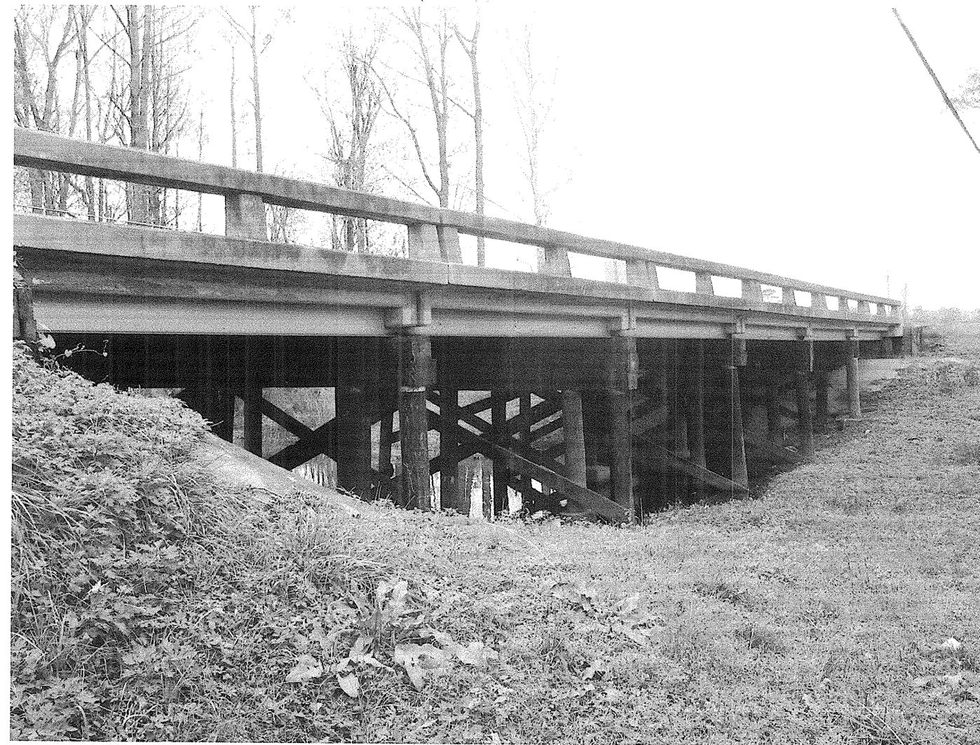
Looking northwest towards End Bent 2
