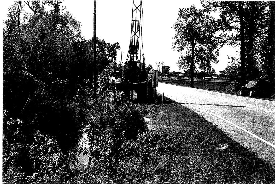
Photograph No. 1: Looking up-station along -L- Rev. from B1-A RL. Drill rig is on B2-A RL.
