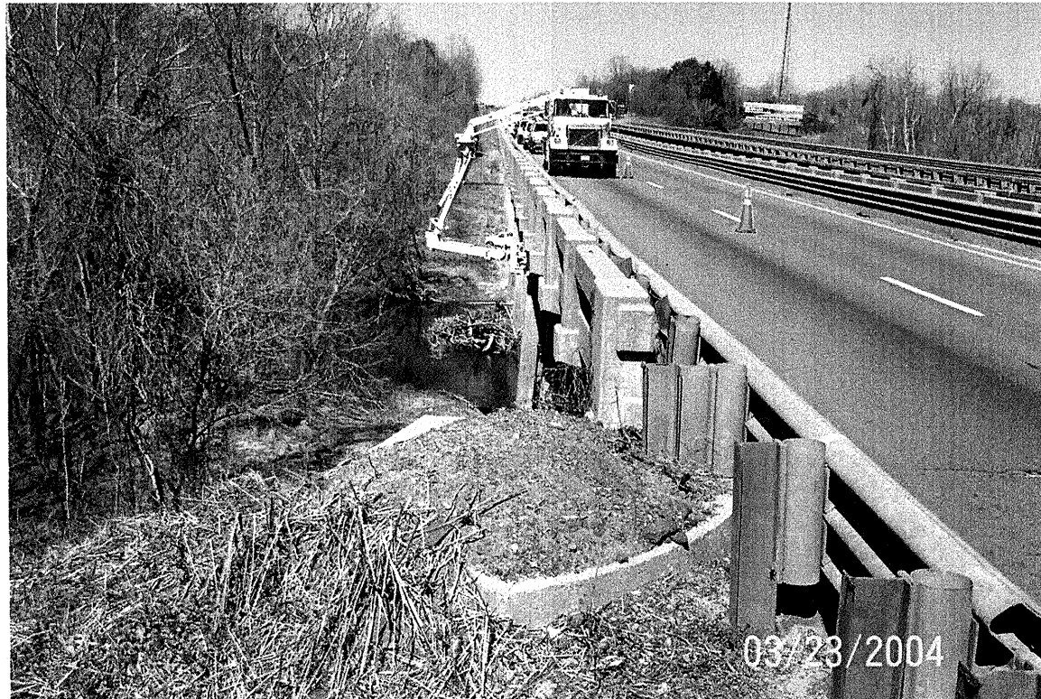
View Approximately 31 Left of -SBL- from End Bent-1 towards End Bent-2
