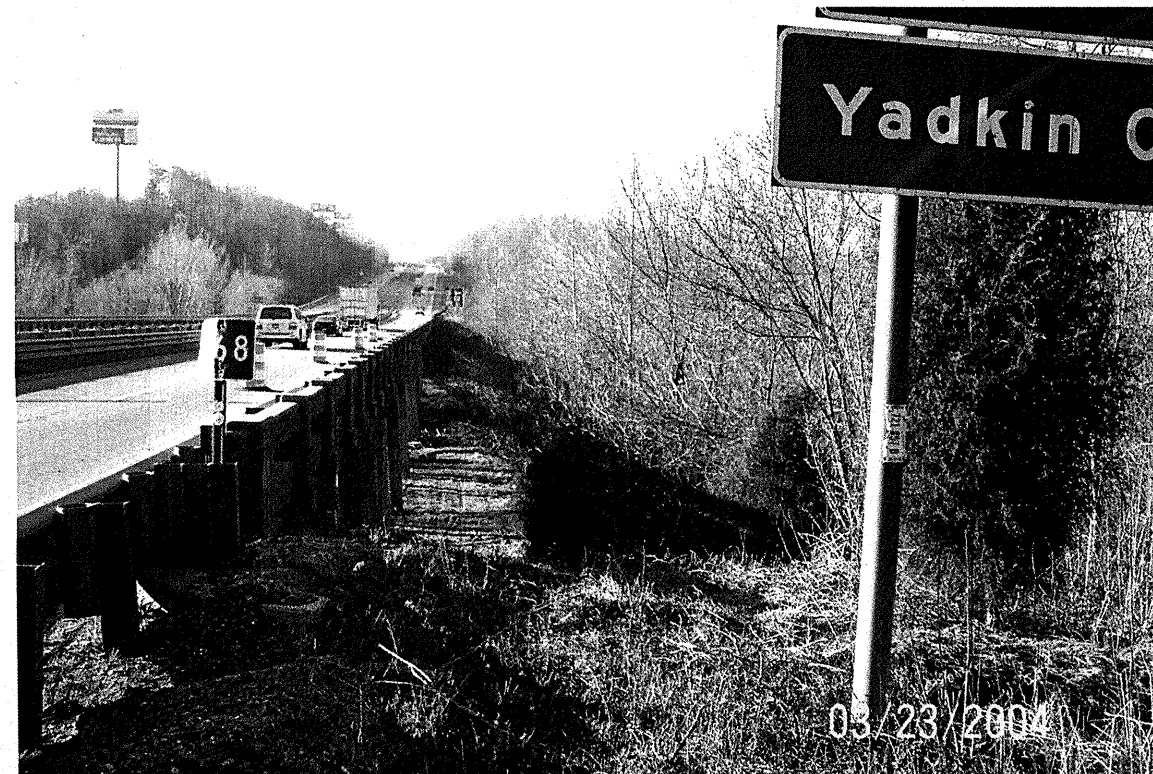
View Approximately 31 Left of -L- from End Bent-2 towards End Bent-1
