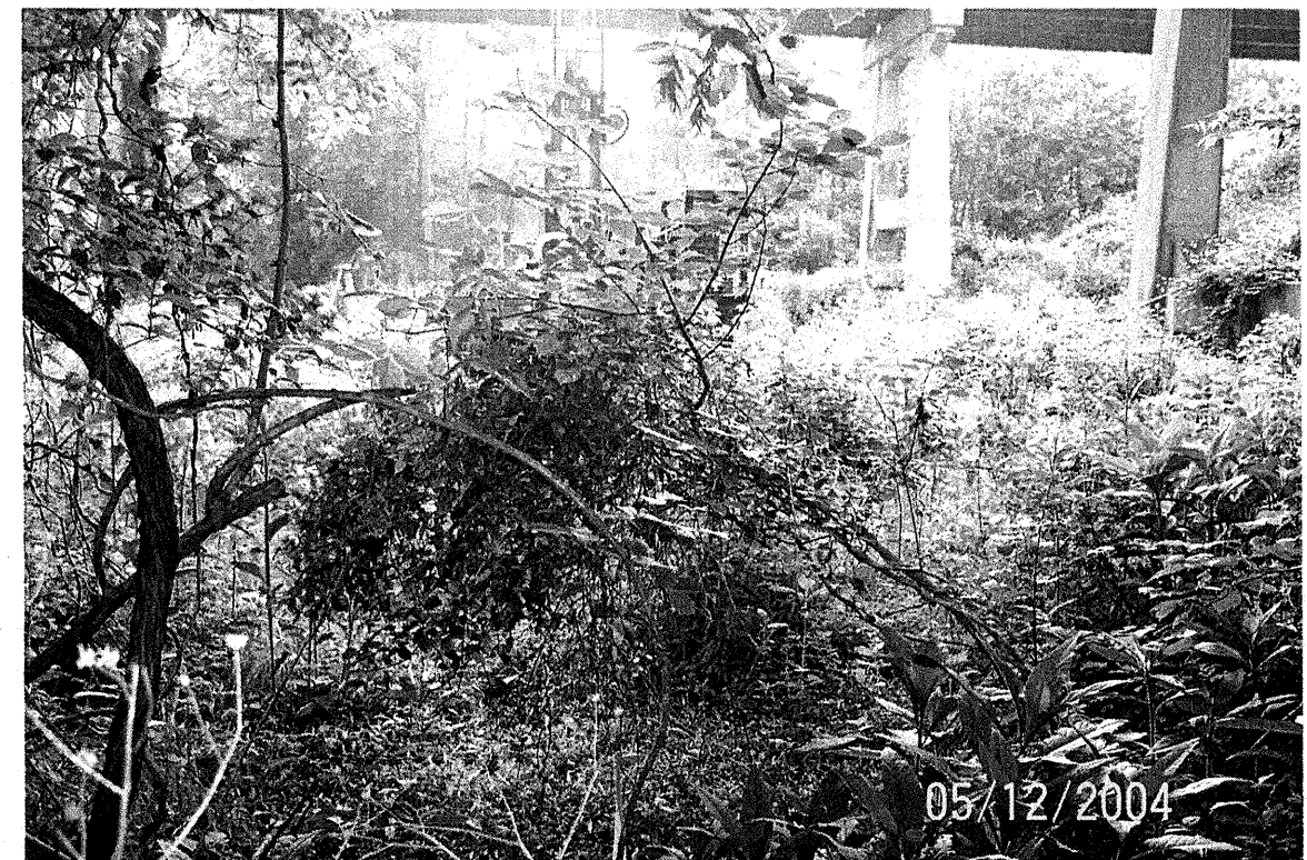
View Along Bent-1 Concrete Span from Left to Right
