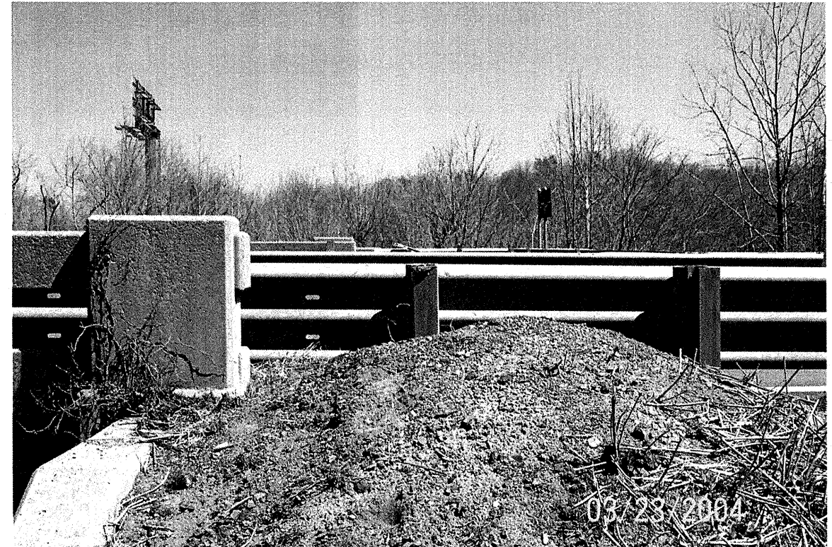
View Along End Bent-1 from Just Left of -SBL- Looking Right
