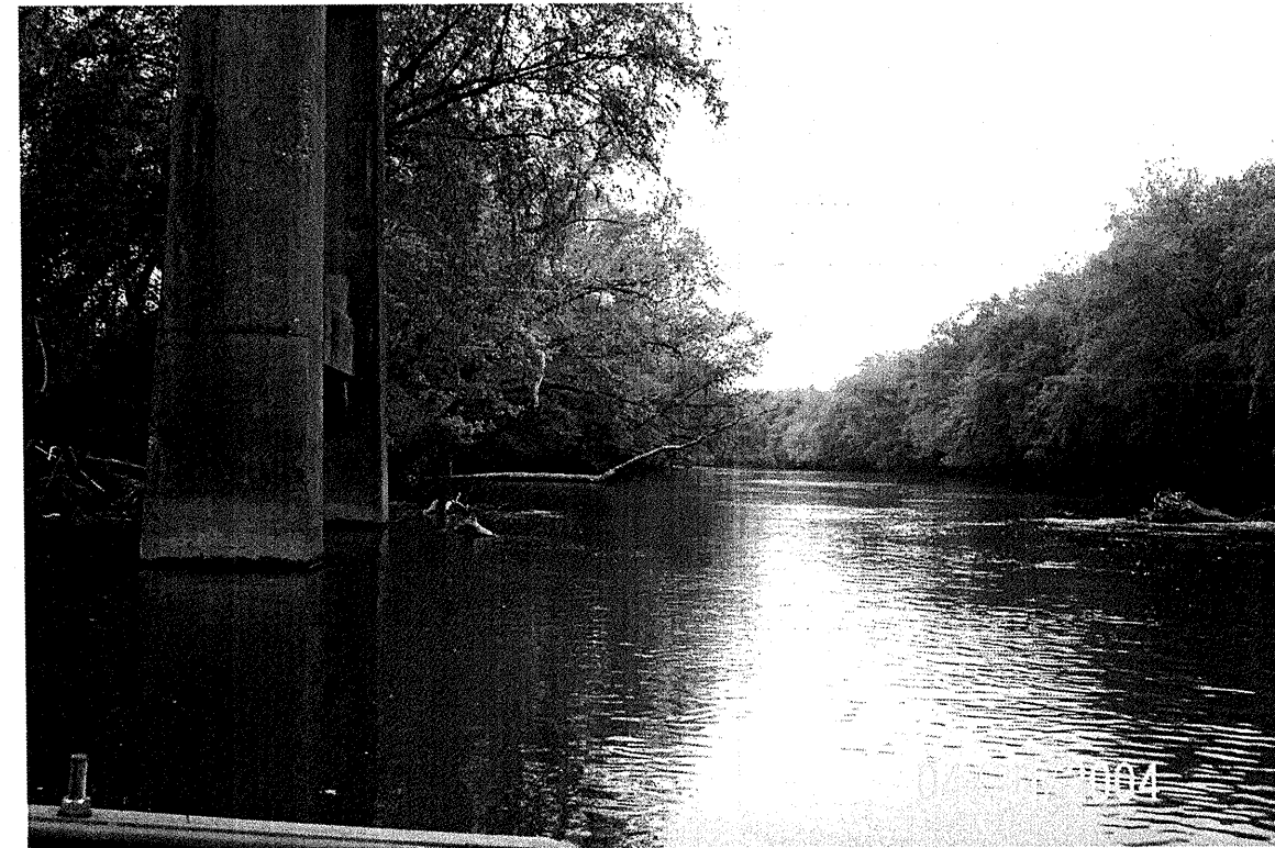
View Along Bent-2 Concrete Span from Right to Left
