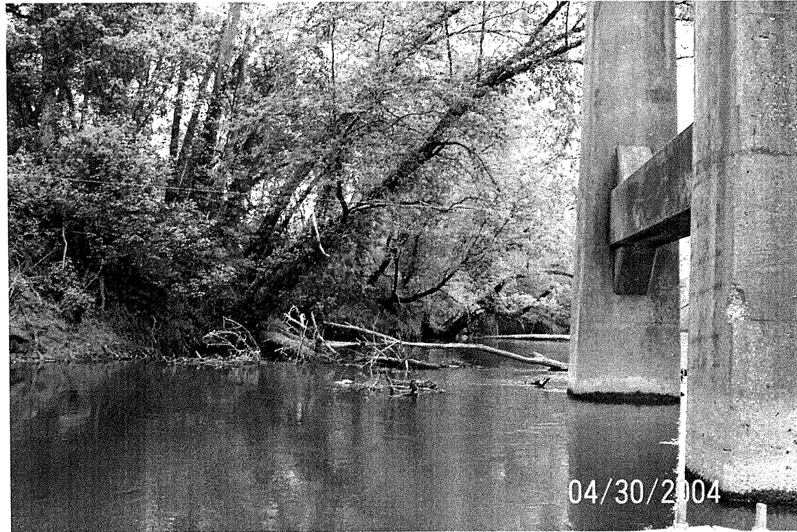
View Along Bent-1 Steel Span from Right to Left
