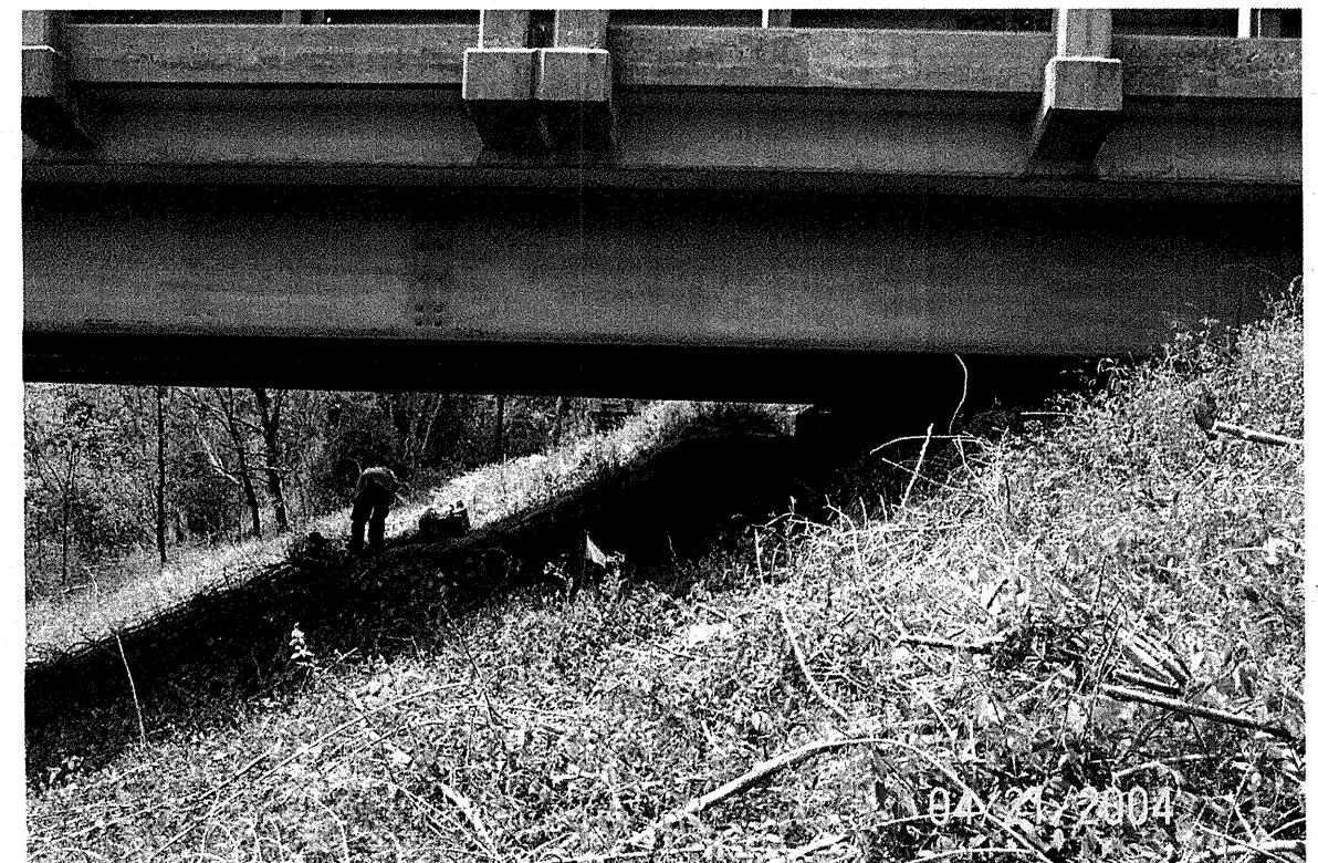
View Along End Bent-2 from Right to Left
