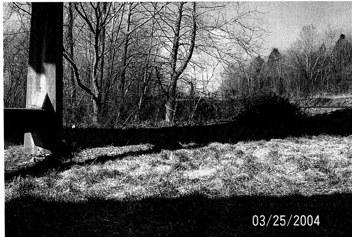
View Along Bent-3 Steel Span/Bent-5 Concrete Span from Right to Left
