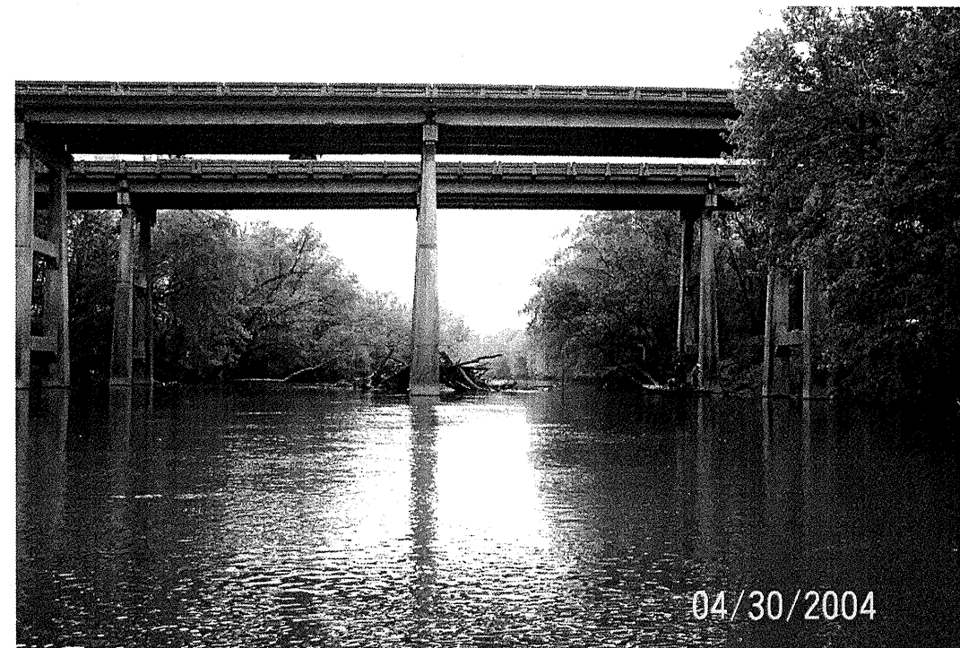
View of Existing Bridges Looking Upstream
