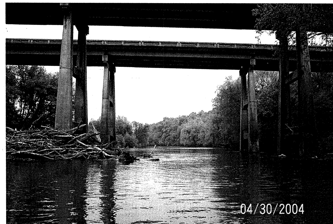
View of Existing Bridges Looking Downstream
