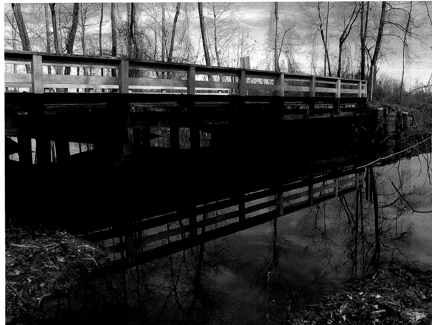
Looking east towards End Bent 2
