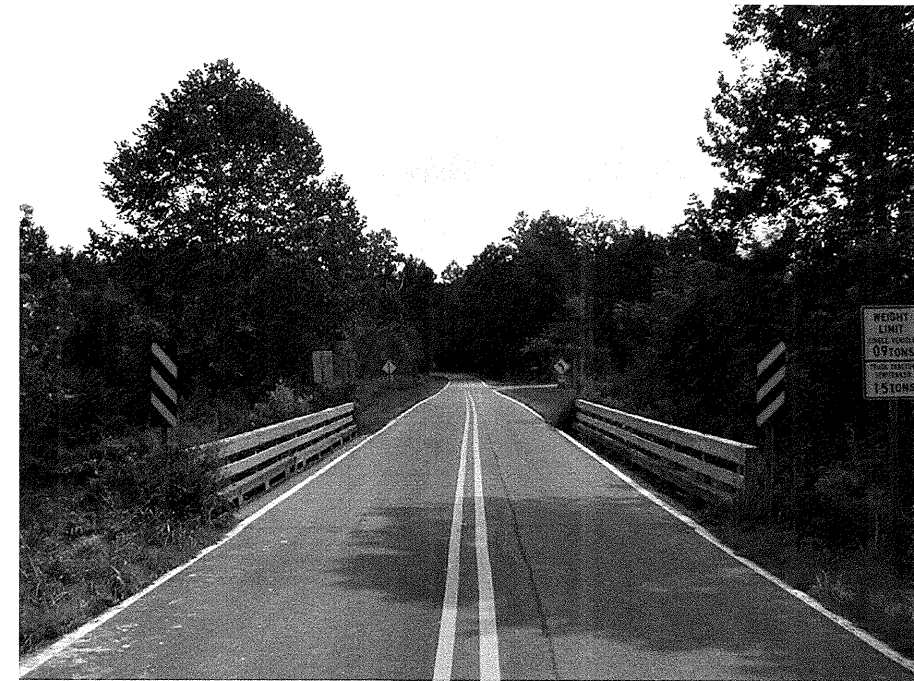
Looking Increasing Station along -L-
