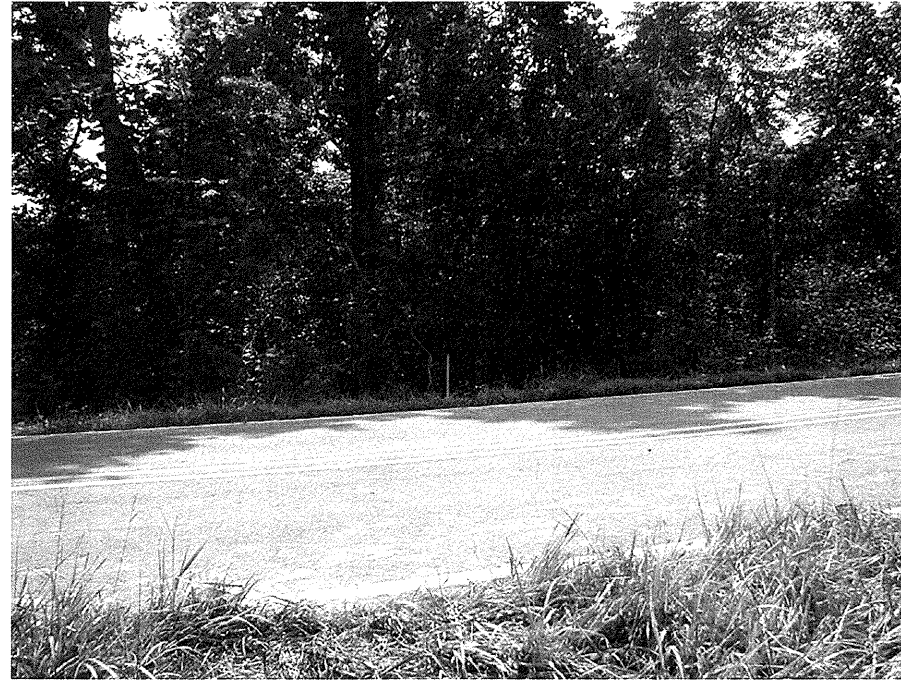
Looking Left to Right along End Bent-1
