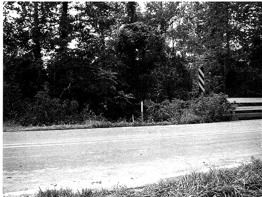
Looking Left to Right along End Bent-2
